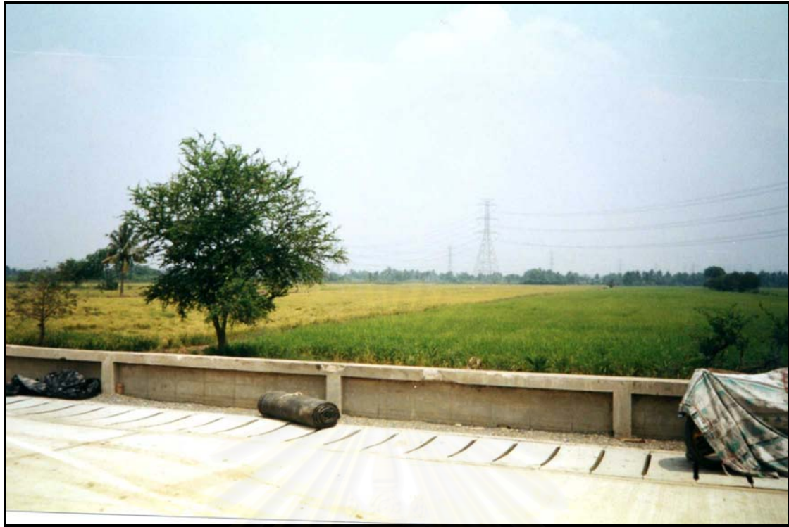
Appendix VI-7 After ground improvement
