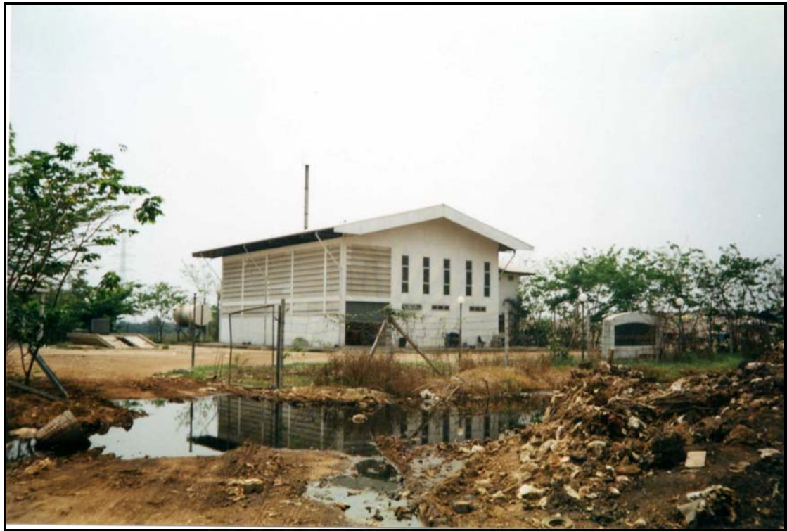
Appendix VI-5 Incineration facility for infectious waste
