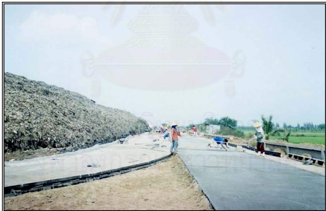
Appendix VI-6 Ground improvement
