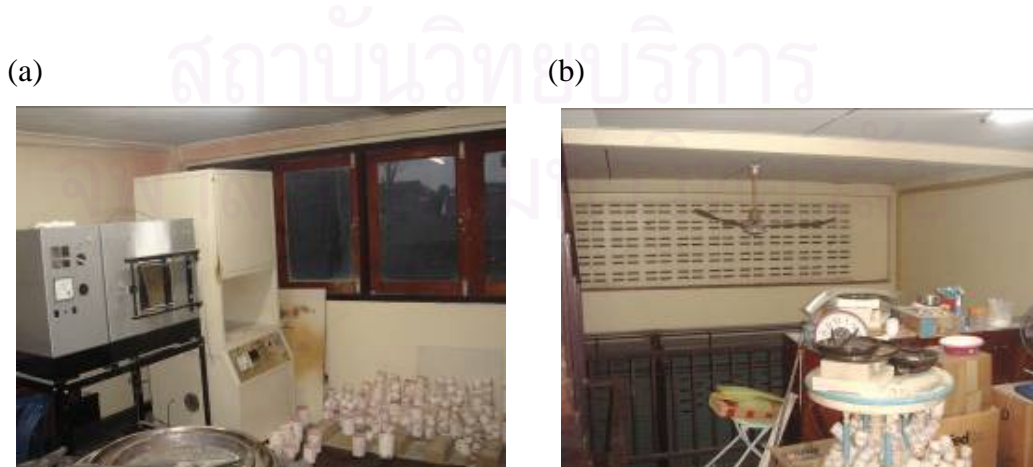
Figure 3.11 (a) Three windows always closed and (b) wall vent holes on the mezzanine.
