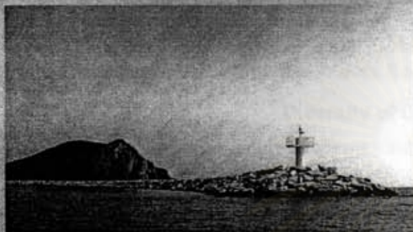
Fig. 1 The 800 m long breakwater located at the Royal Thai Navy, Sattahip, Chonburi Province
