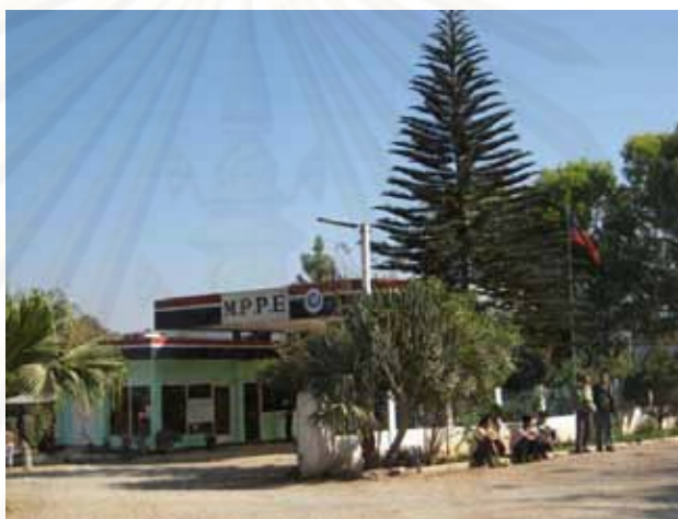
Figure 5: M.P.P.E Gas Station in Shan State in urban area of Taunggyi
