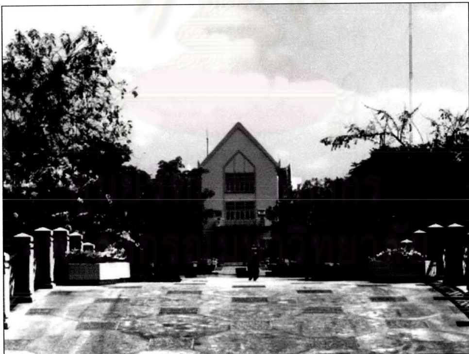
B-4: Building site in Queen Sirikit Park
