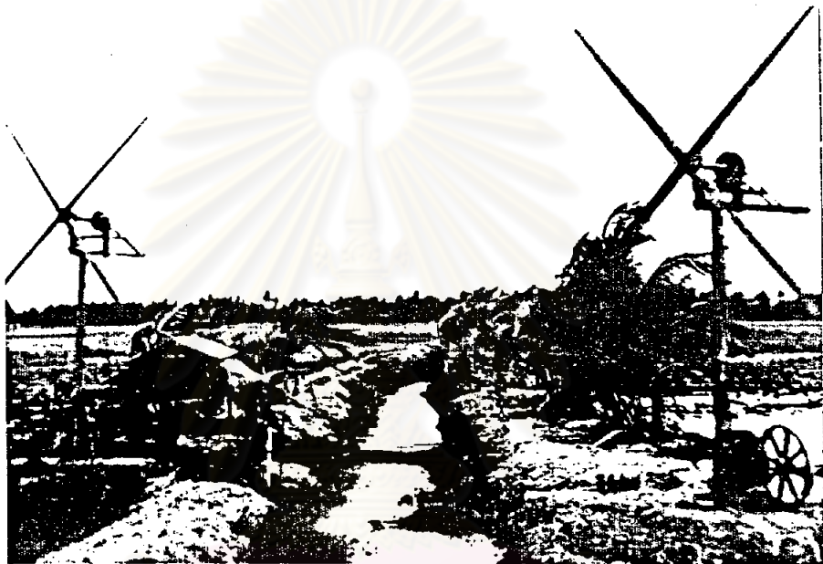
Fig.B.2 High speed wooden rotor windmill
