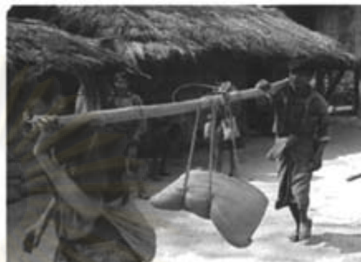
Figure 31: Villagers contribute their labor to repair a damaged irrigation canal (Food security project).
