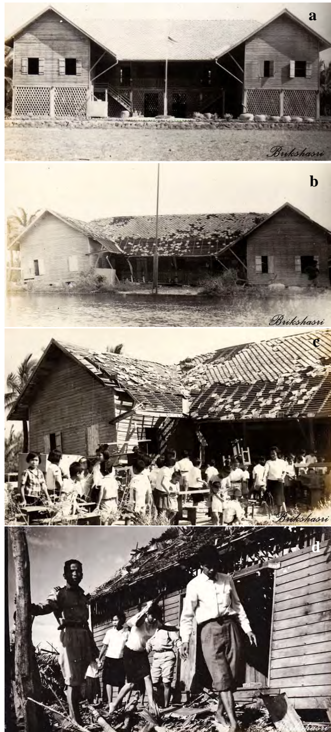
Figure 2.12 Comparing pictures of school's building "before and after" which resulted from Harriet in 1962. Picture a) showing the two floors building before the storm event and b) the collapsed building after the storm event. c) Students are removing the desks out of the collapsed building and d) the official's governments are surveying the damage from Harriet. (pictures from http://www.gotonakhon.com )
