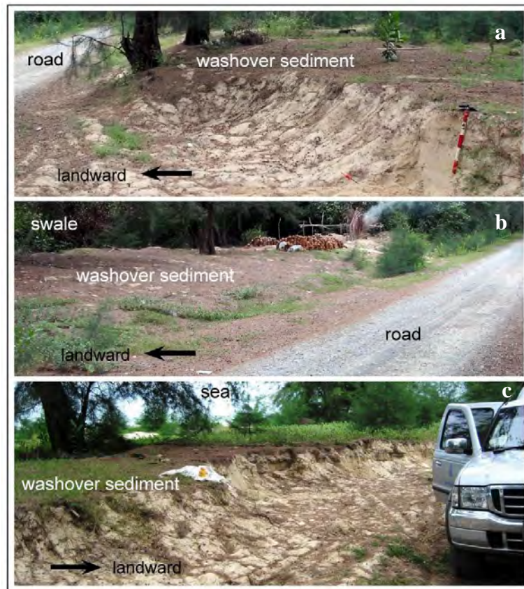
Figure 4.48 a) and c) Road cut profile of washover deposit along the road behind beach. b) The remaining washover sediment penetrated into a swale. Picture taken location is indicated in Figure 4.40.
