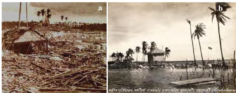
Figure 2.11 Damage from Tropical storm Harriet in 1962 at Laem Talumphuk sand spit. Picture a, b show destroyed houses and coconut tree along the shoreline of LT sand spit. (pictures from http://paipibat.com and http://www.gotonakhon.com )
