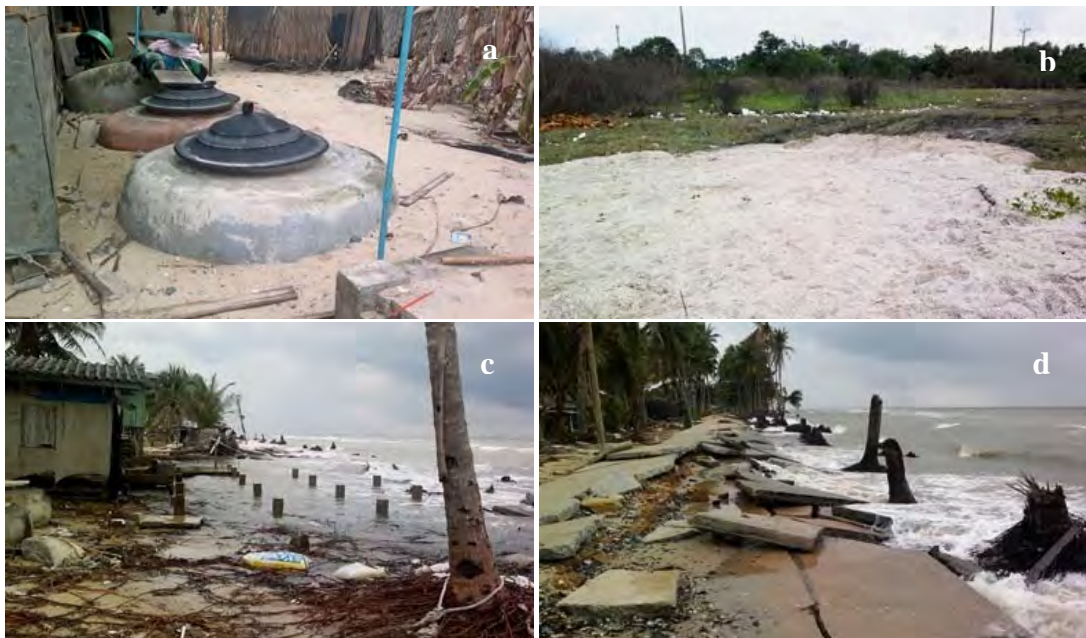
Figure 2.25 Washover deposits and damage from storm surge at Laem Talumphuk, Nakhon Si Thammarat province on 25 December 2011. a) Washover deposit thick 60cm in the village and b) washover sediment deposit far 50m from shoreline. c) and d) Destroyed house and road . (pictures from http://www.oknation.net/blog/nn1234/2012/01/02/entry-1 )
