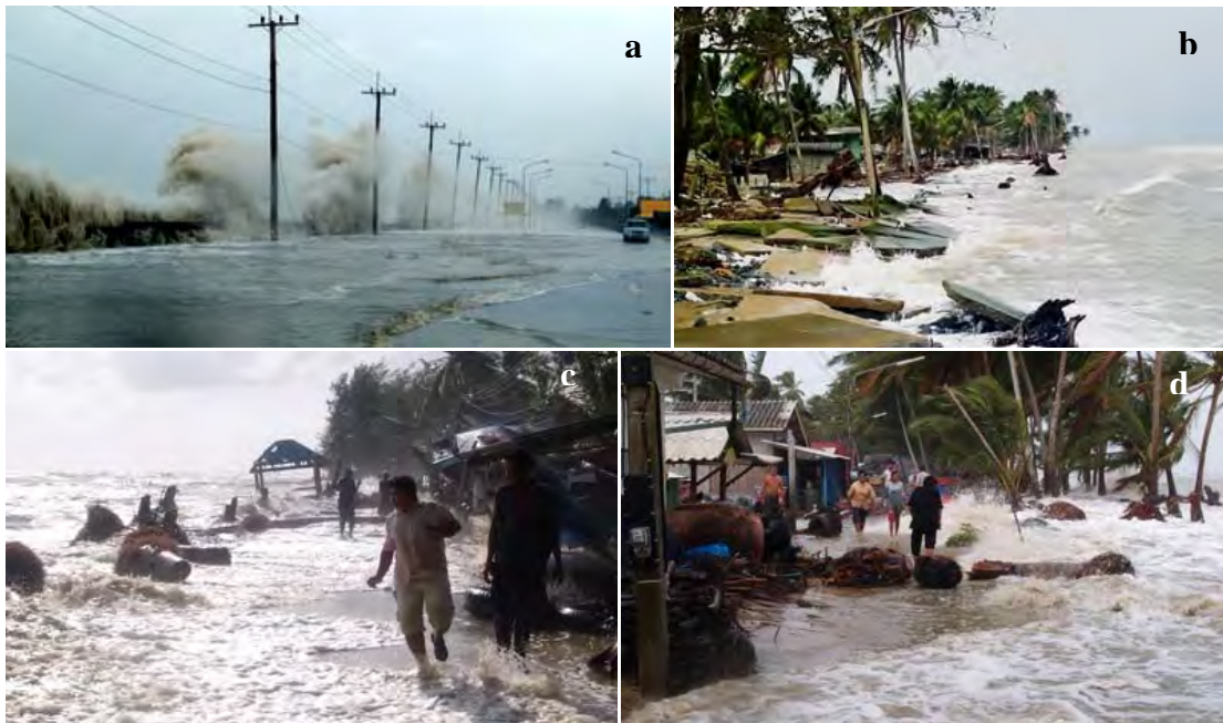
Figure 2.24 Storm surge and overwash flow at Laem Talumphuk, Nakhon Si Thammarat province on 25 December 2011. a) Wave splashing high 6-7 m during the attack at the seawall. b) Destroyed road and house along the shoreline. c) and d) Overwash flows are flooding in to the village near shoreline. (picture a), c), and d) from http://www.mana.co.th , b) from http://www.oknation.net/blog/nn1234/2012/01/02/entry-1 )
