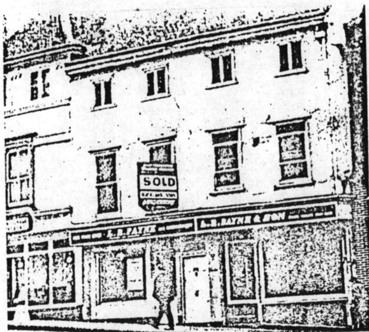
▲ No. 12 Thames Street was in poor condition; it has now been renovated, with new shops at ground level and upper floors let as offices B & C
