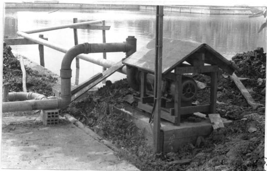
FIGURE 4.3 CENTRIFUGAL PUMP AND PIPING
