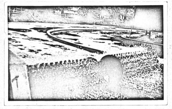
SHOWS THE OXIDATION DITCH WITH ROTATING CAGE ROTOR AT TAK HOSPITAL
