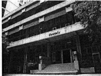
Figure 2b – Building 4 of the Faculty of Arts, Chulalongkorn University, where the Art Theatre was located
