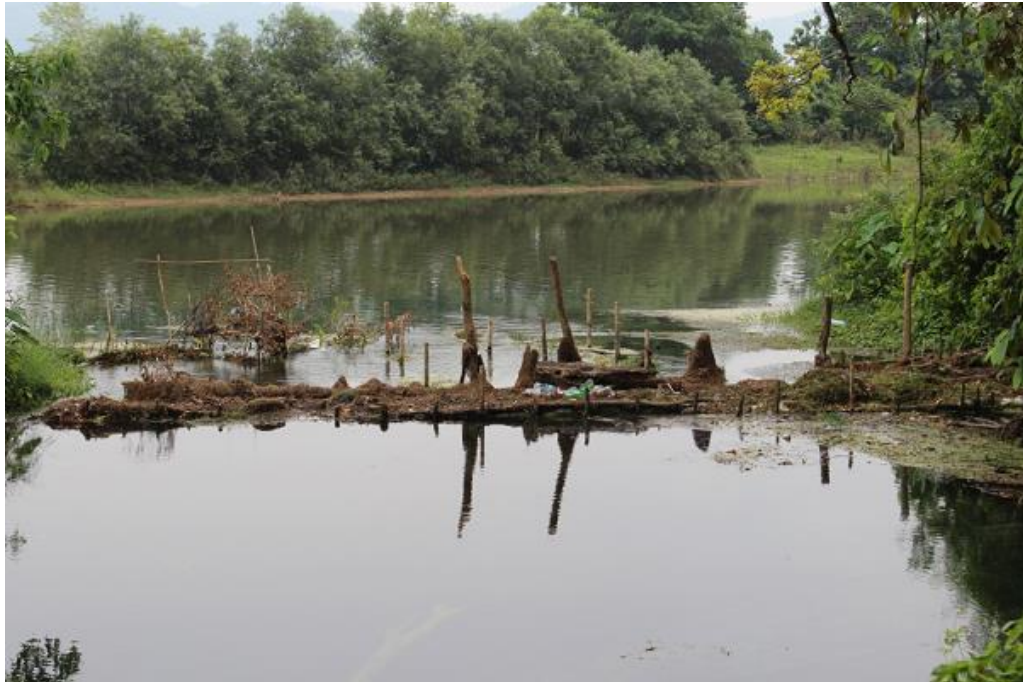
Figure 4.2 Wood weir in Vang Vieng District as of 6 th June 2014
