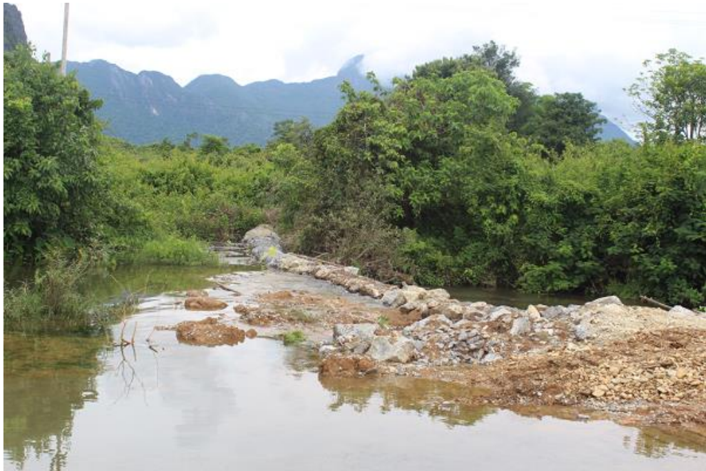
Figure 4.3 Traditional weir or Native weir (gabion weir) in Na MOUNG village 2014
