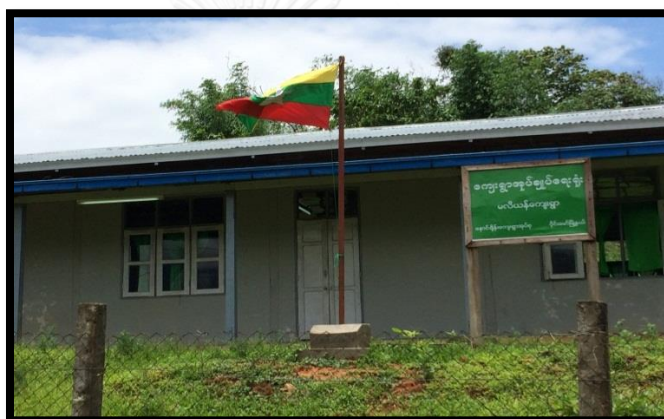
Photograph (8) Village Administration office in Maliyang Relocation village
