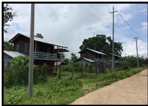
Photograph (5) Houses in Relocation Villages
