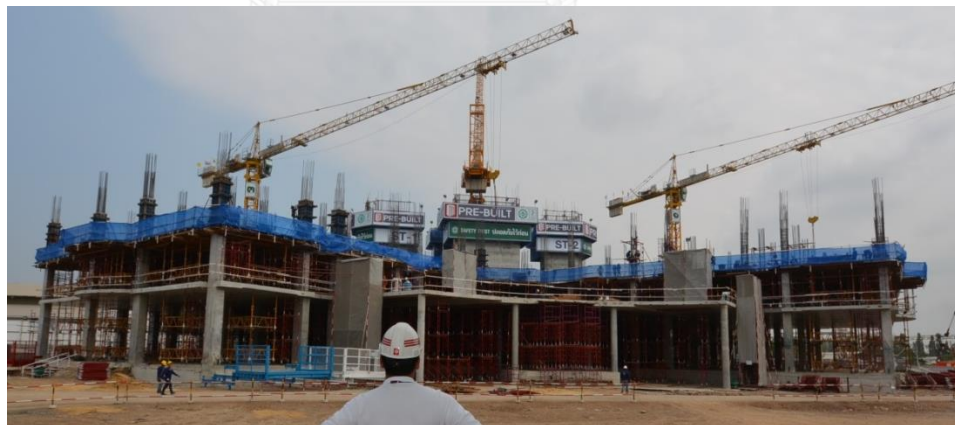
Figure 7.5 All of tower cranes on the site
