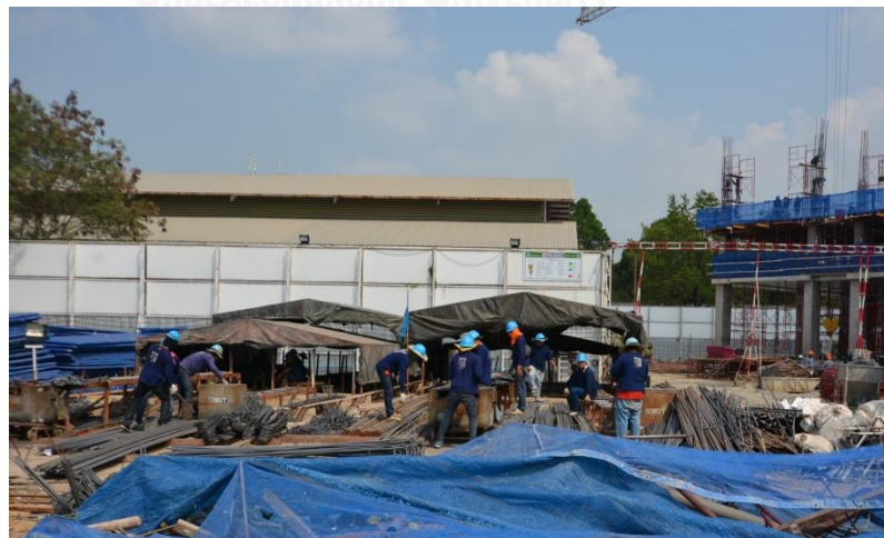
Figure 7.14 Steel yard on the site
