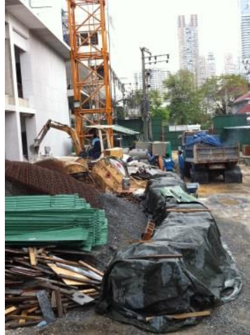
Figure 4.10 Laydown area on the construction site
