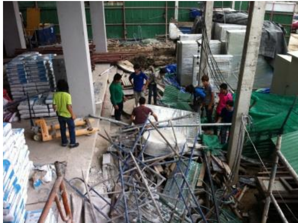
Figure 4.13 Stock yard where the tower crane cannot reach
