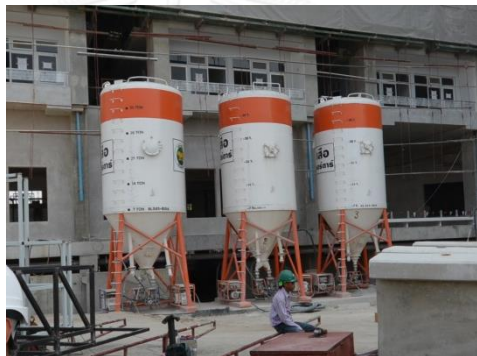
Figure 4.5 Mobile cement plant
