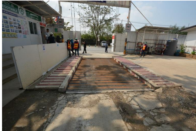
Figure 7.18 Washing yard for tires of trucks on the site
