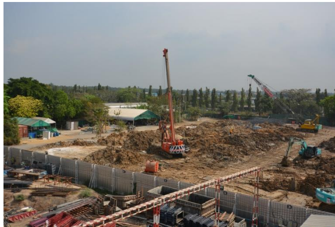
Figure 7.4 Nearby environment of the construction site
