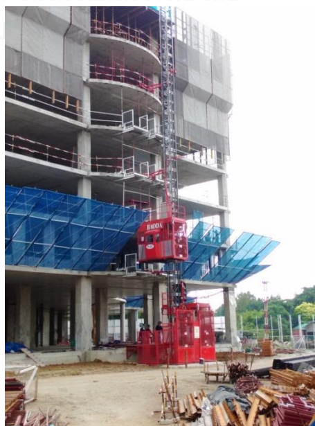
Figure 7.7 Double cages passenger lifts on the site
