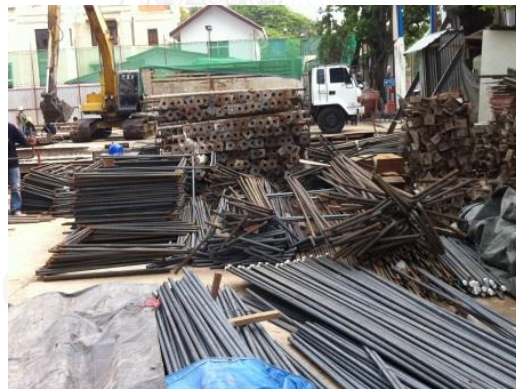
Figure 4.9 Steel yard on the construction site
