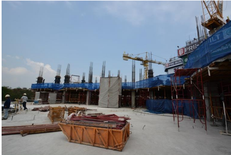
Figure 7.2 Clean work area and the protection
