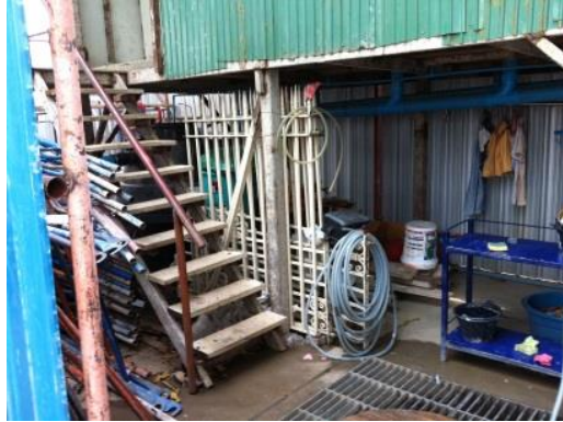
Figure 4.7 Toilet on the construction site
