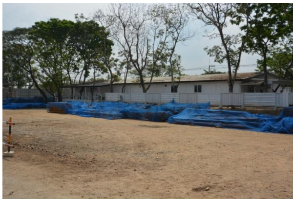
Figure 7.15 Laydown area on the site
