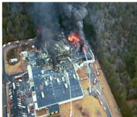
Polyethylene dust explosion- west pharmaceuticals (6 fatalities)
