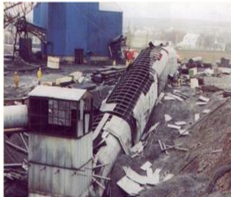
Methane triggered coal dust explosion- westray, coal mine (26 fatalities)
