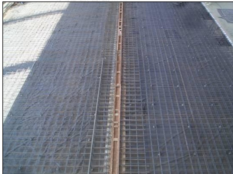
Figure 3.7: Slab-on-grade of Project- B under the Construction
