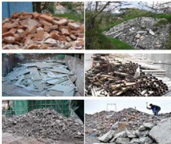
Figure 2.1 Construction Waste in Current Practice
