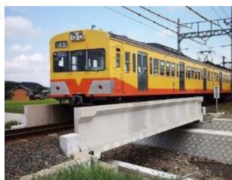
(ข) Kayogawa UFC Railway Bridge
