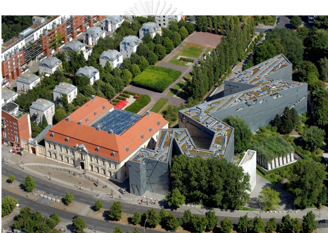
Figure 2. 13 Existing structure versus the New building of Jewish museum © Guenter Schneider
