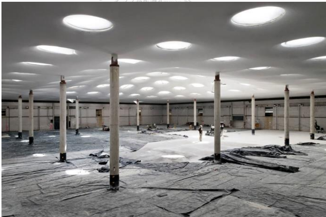
Figure 2. 26 Construction phase of Städel Museum © Schneider+Schumacher
