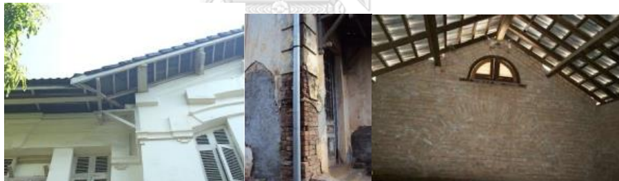
Figure 2.13 The use of brick and some part of wooden roof structure
