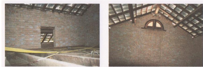
Figure 4.14 Roof structure of existing building
