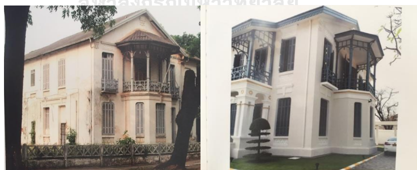
Figure 2.38 Before and after the restoration of the Embassy of Brunei Darussalam in Vientiane, Lao PDR (Source from the Embassy of Brunei Darussalam in Vientiane, Lao PDR, 2014)
