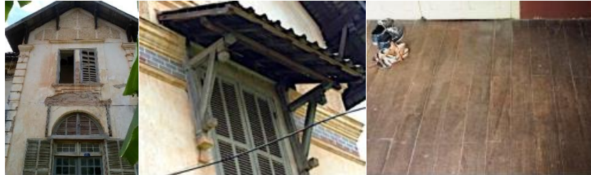
Figure 2.12 Pictures of stucco design above window, wooden strut and wooden floor
