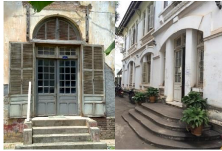
Figure 2.9 Pictures of the entrance doors of Colonial building
