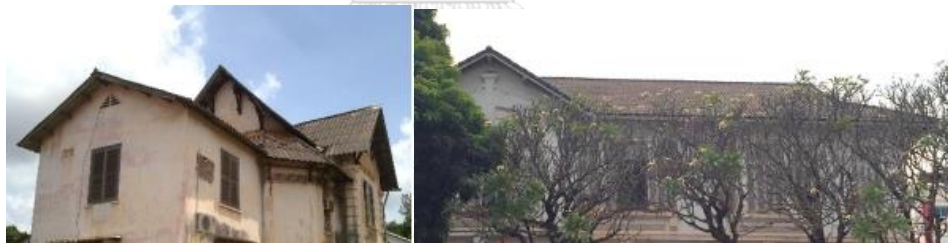
Figure 2.8 Pictures of the use of Din Kho roof tile of Colonial building
