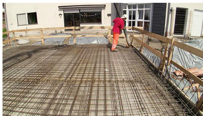
Figure 1.1: Casting method applied in real constructions
