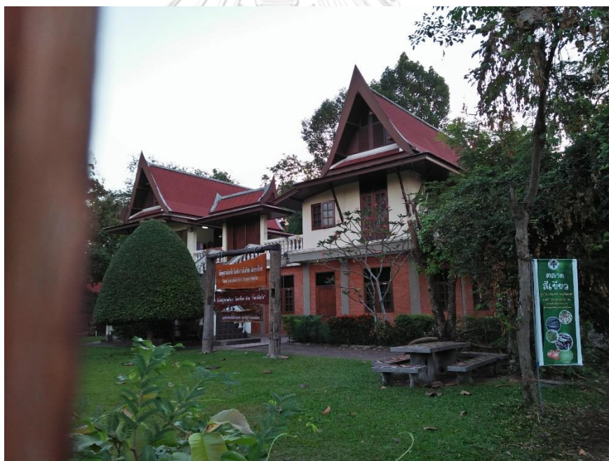
Figure 13 Kud-Chum District Hospital (photo taken by Yan-Ting Huang.)
