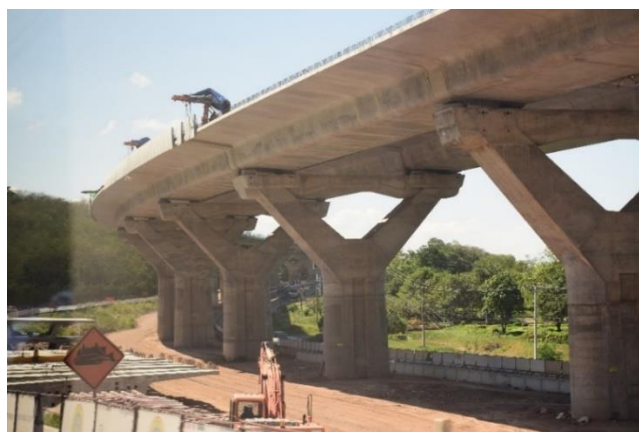
Figure 2.1 An elevated highway construction project
