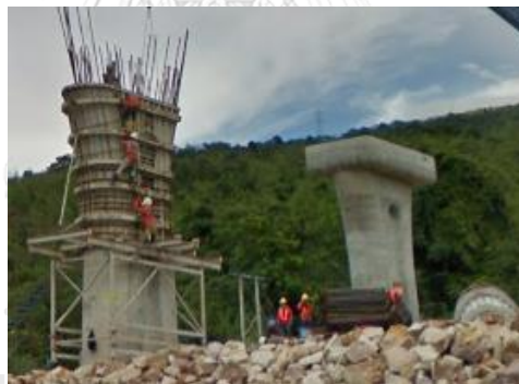
Figure 3.7 Fabricated formwork for top column P11
