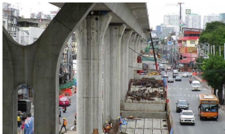
Figure 2.6 Piers in an elevated railway construction project
