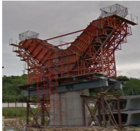
Figure 3.9 Fabricated formwork for Y-shape column P13
