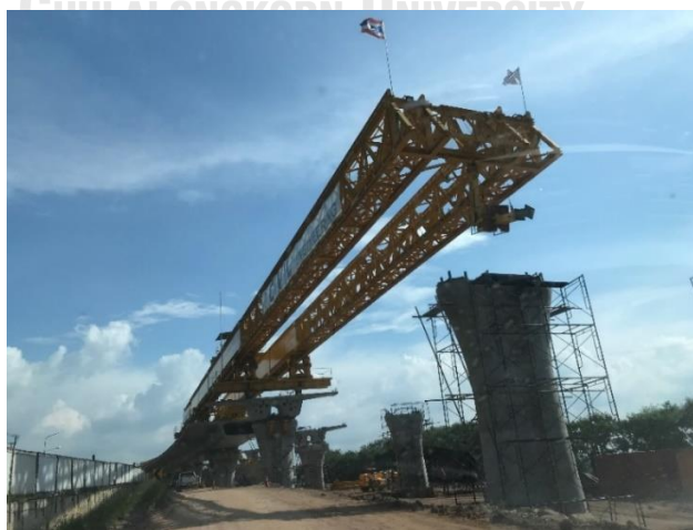
Figure 2.3 Pre-cast segment erection with launching gantry (LG)
