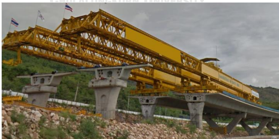
Figure 3.10 Launching gantry for the viaduct precast segment erection
