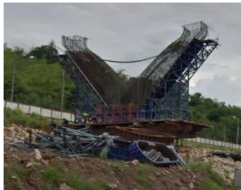
Figure 3.7 Fabricated formwork for top column P11
