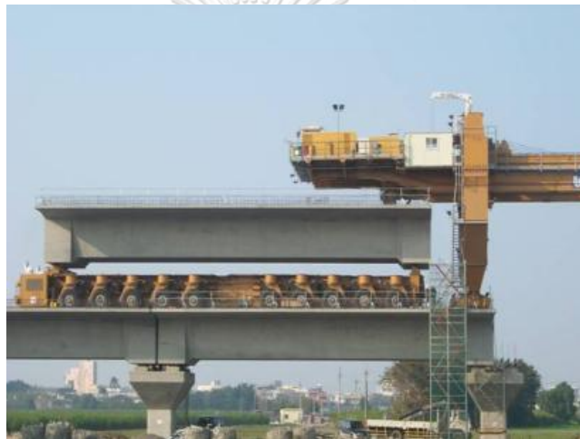
Figure 2.4 Full Span Precast Method (FSPM)
