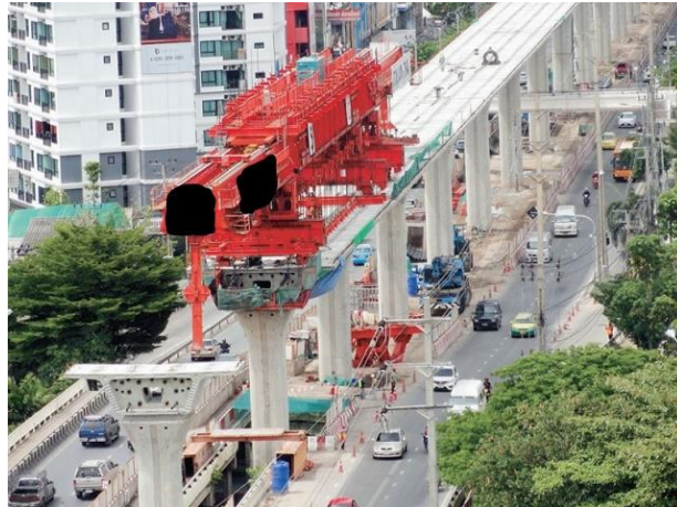
Figure 2.5 Straight-line performance of launching gantry
