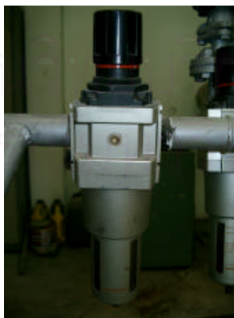
Figure 4.7 Filter and Pressure Regulator Set
