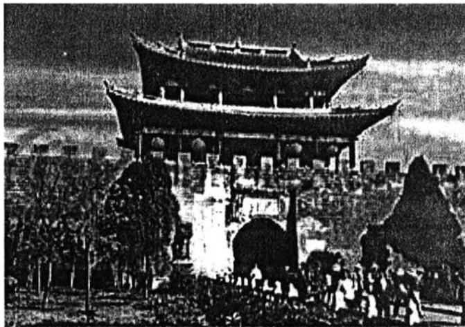
2.5, Dali Old Town gate and wall Photo Source: Dali Luyou Xinxigang
