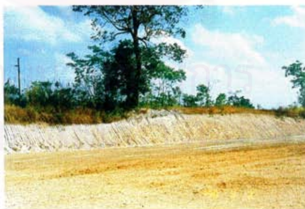
Figure 2.18 Residual and colluvium-elluvium deposit of sandstone, siltstone
