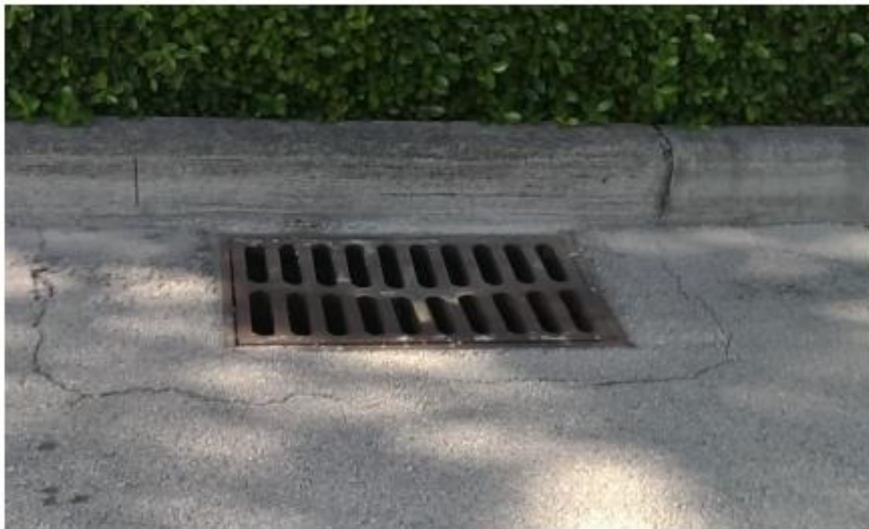
Figure B-2: Type 3 - Grate inlet
