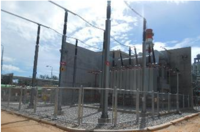
Figure 36 Transformer installation (Project D monthly reports)
