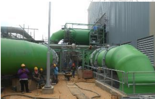
Figure 42 Cooling water pipes installation (Project D monthly reports)
