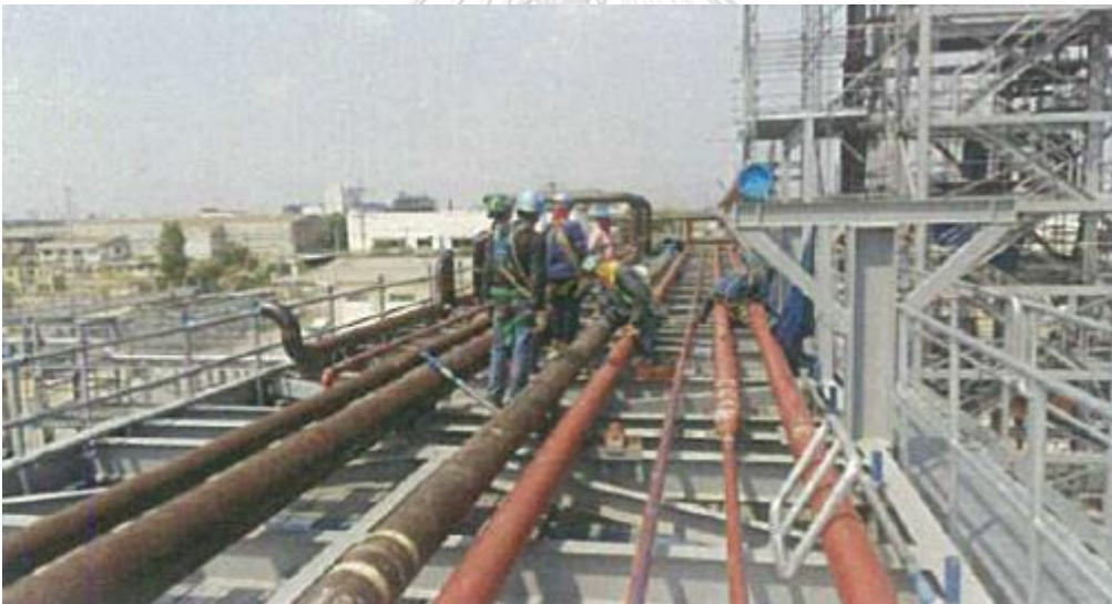
Figure 40 Piping system installation (Project B monthly reports)
