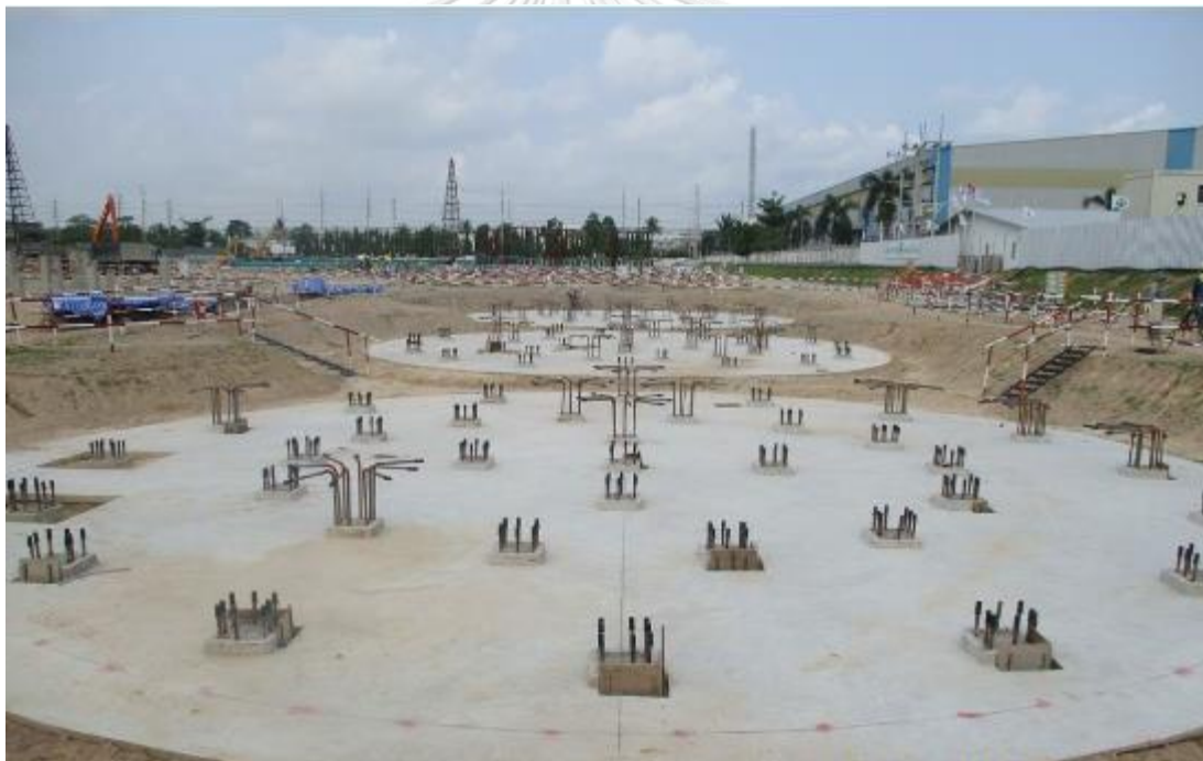
Figure 17 Tanks foundation lean concrete pouring (Project A monthly reports)
