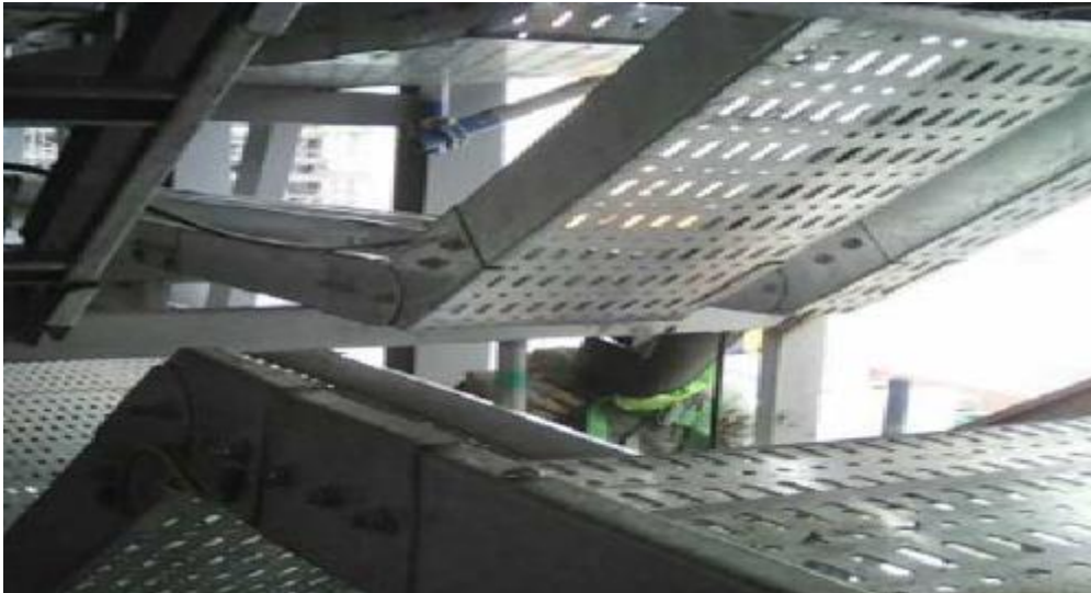
Figure 45 Cable tray installation (Project B monthly reports)
