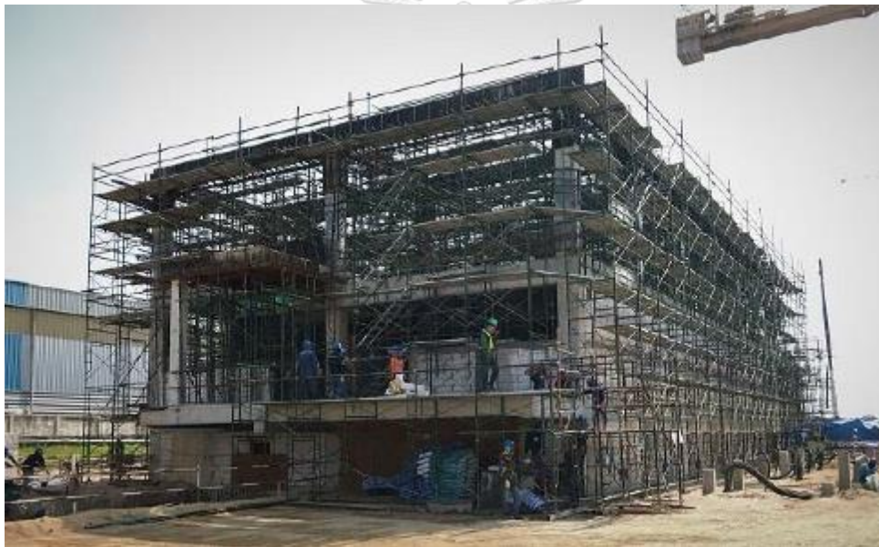
Figure 21 Central control building installation (Project A monthly reports)
