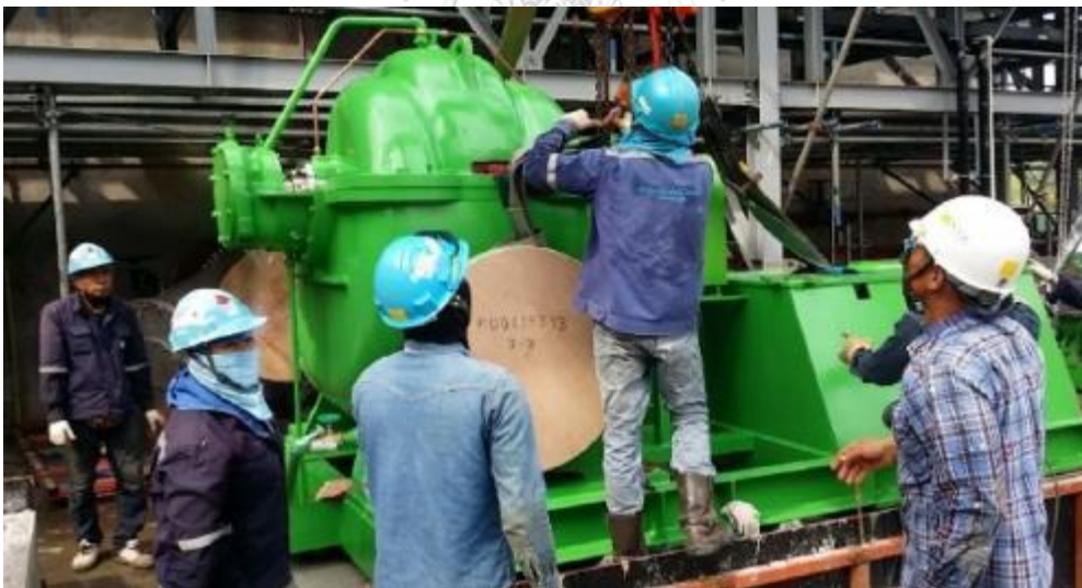
Figure 35 Cooling water pumps installation (Project B monthly reports)
