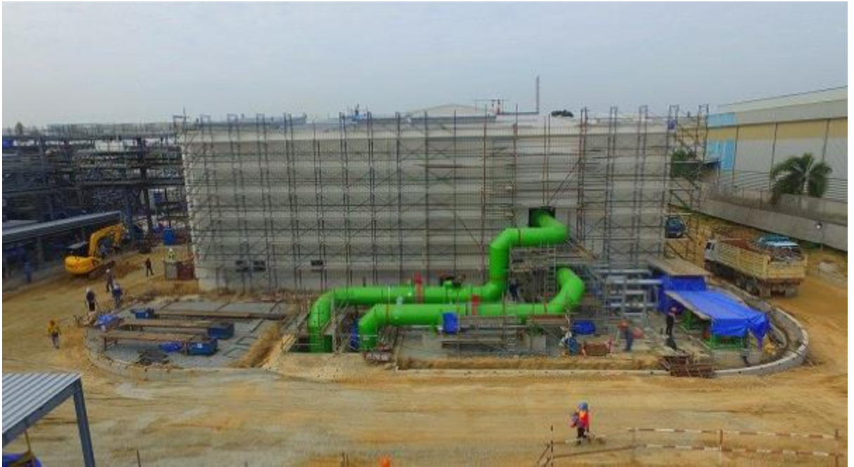
Figure 41 Cooling water pipes installation (Project A monthly reports)
