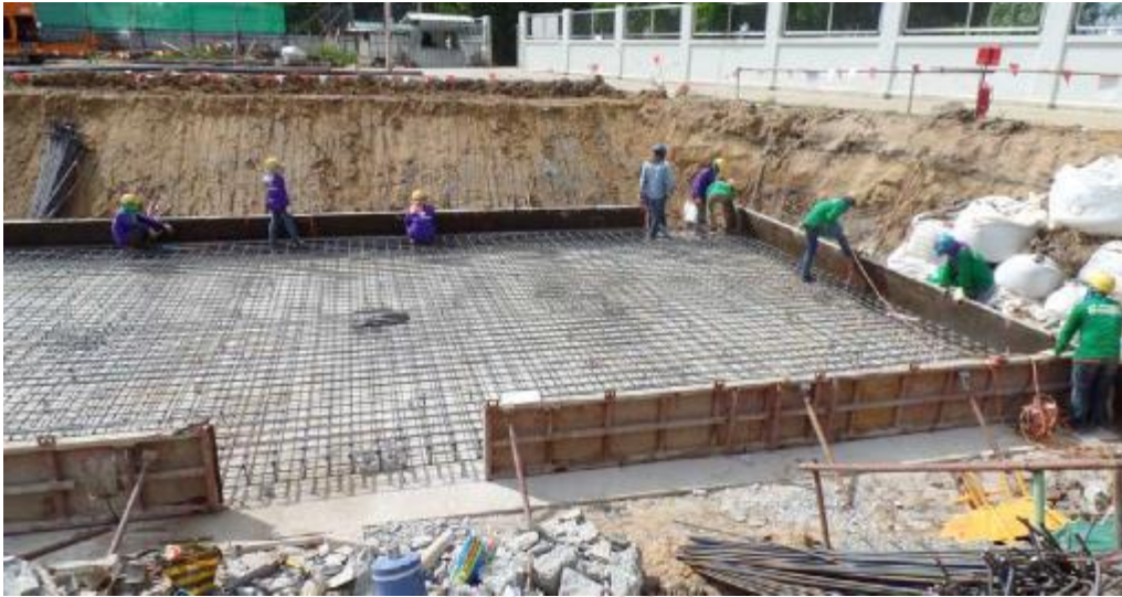
Figure 25 Water pond construction (Project B monthly reports)
