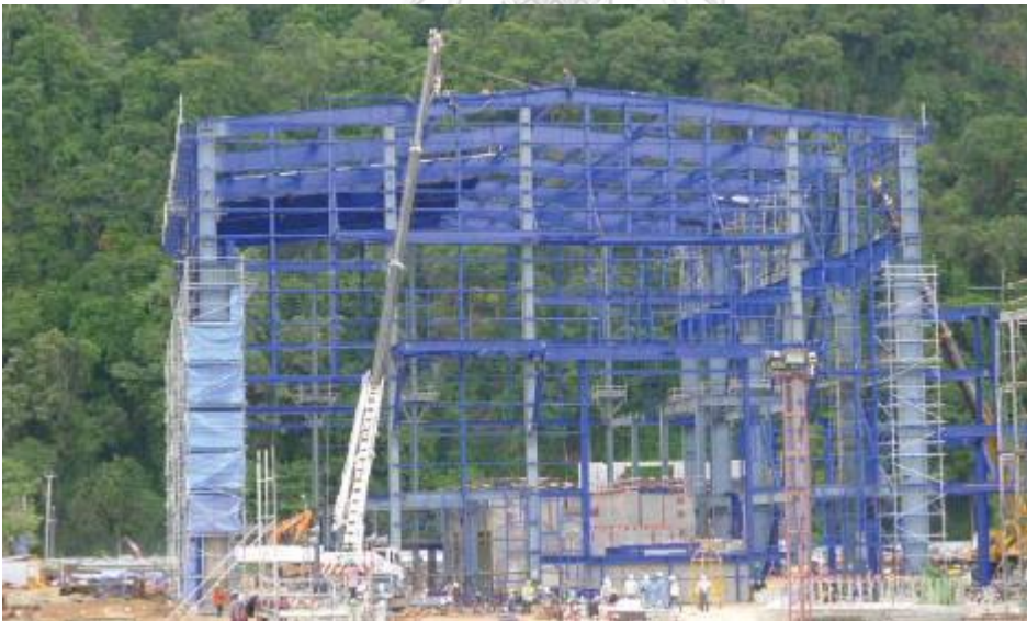
Figure 23 Turbine building installation (Project D monthly reports)
