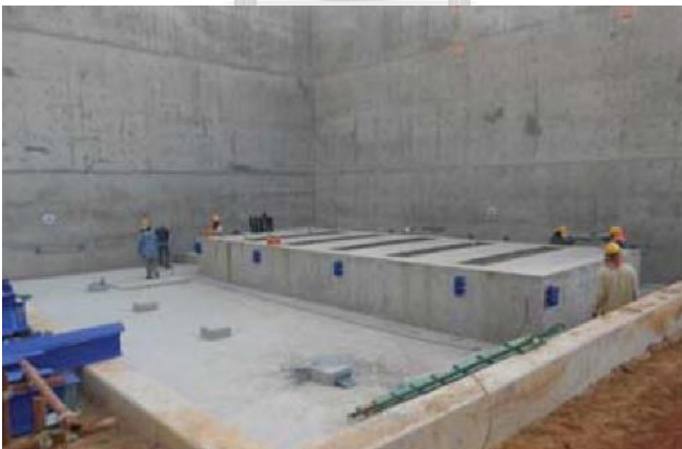
Figure 20 Transformer foundation after concrete pouring (Project D monthly reports)
