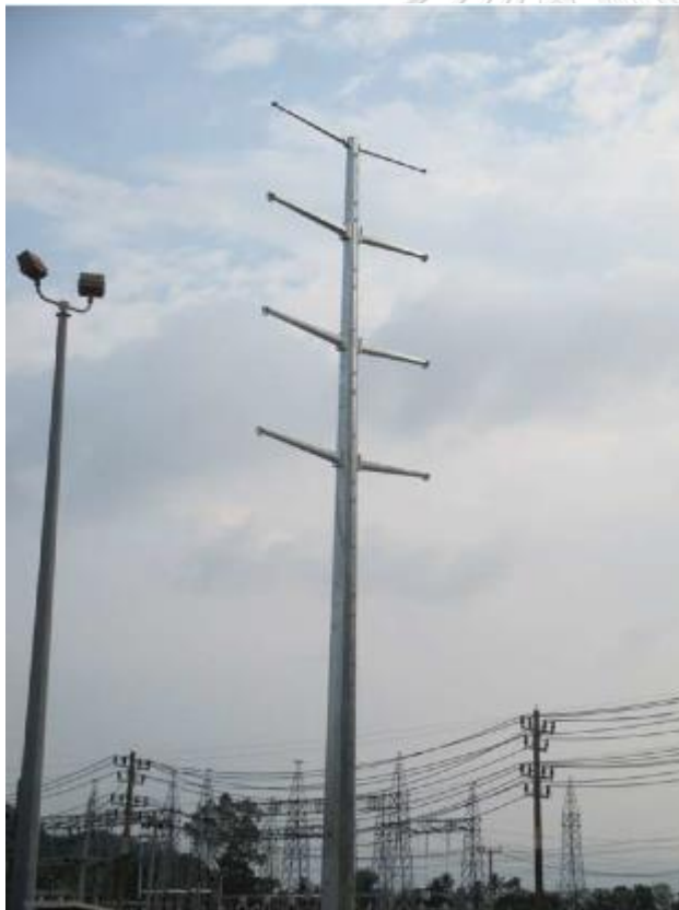
Figure 47 Transmission line installation (Project D monthly reports)
