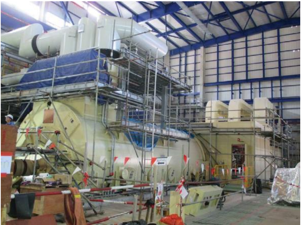
Figure 27 Gas turbine and generator erection (Project D monthly reports)
