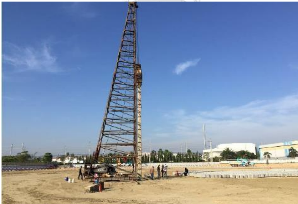
Figure 16 Piling works (Project A monthly reports)
