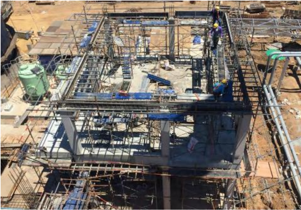
Figure 22 Water treatment building installation (Project C monthly reports)
