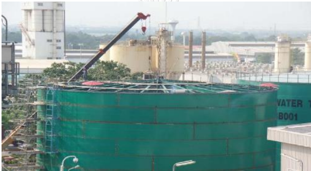
Figure 32 Water tanks installation (Project B monthly reports)
