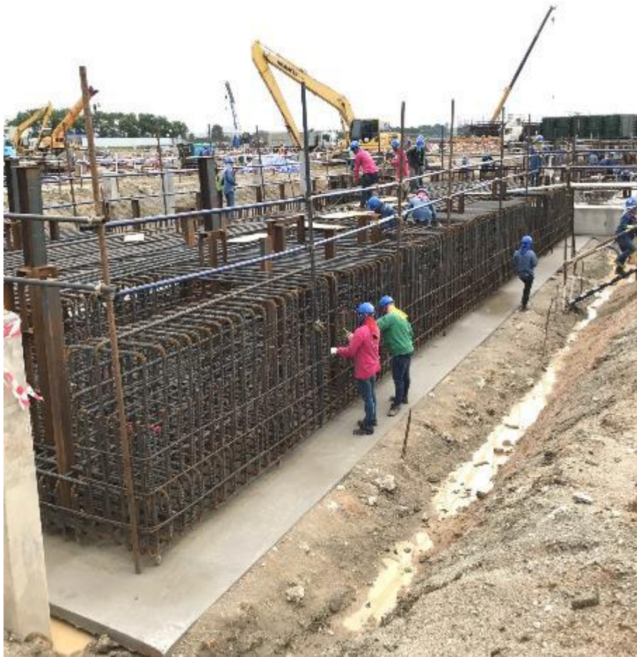
Figure 18 Gas turbine foundation rebar works (Project A monthly reports)
