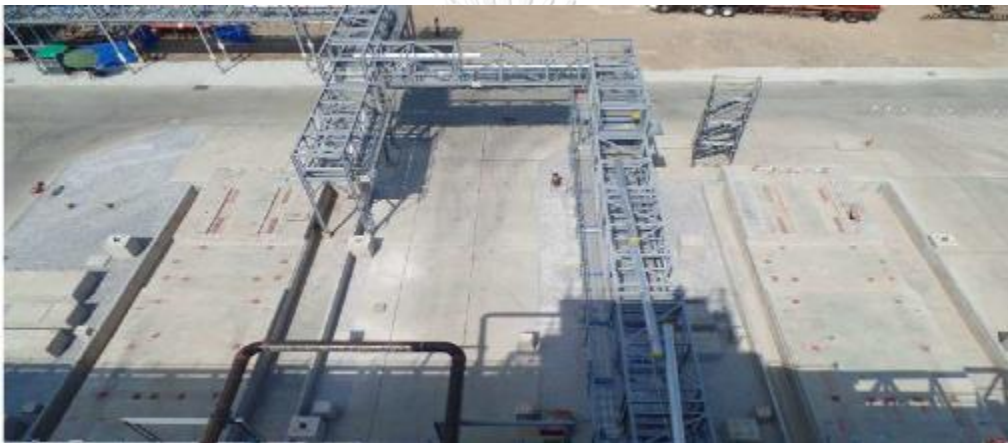
Figure 24 Pipe rack and pipe bridges installation (Project B monthly reports)
