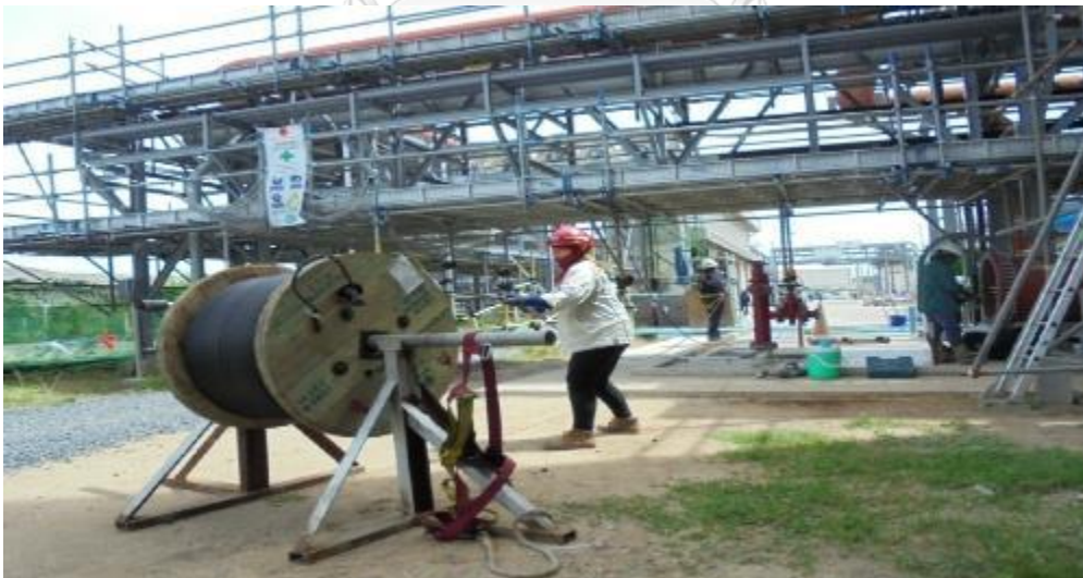
Figure 46 Cabling work (Project B monthly reports)
