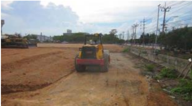
Figure 15 Site preparation works (Project C monthly reports)
