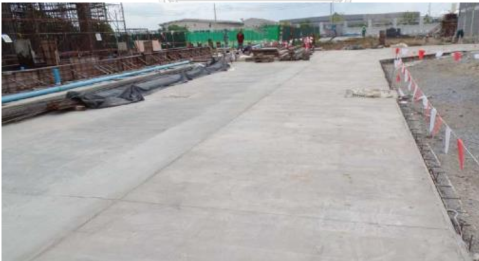
Figure 26 Road construction (Project B monthly reports)
