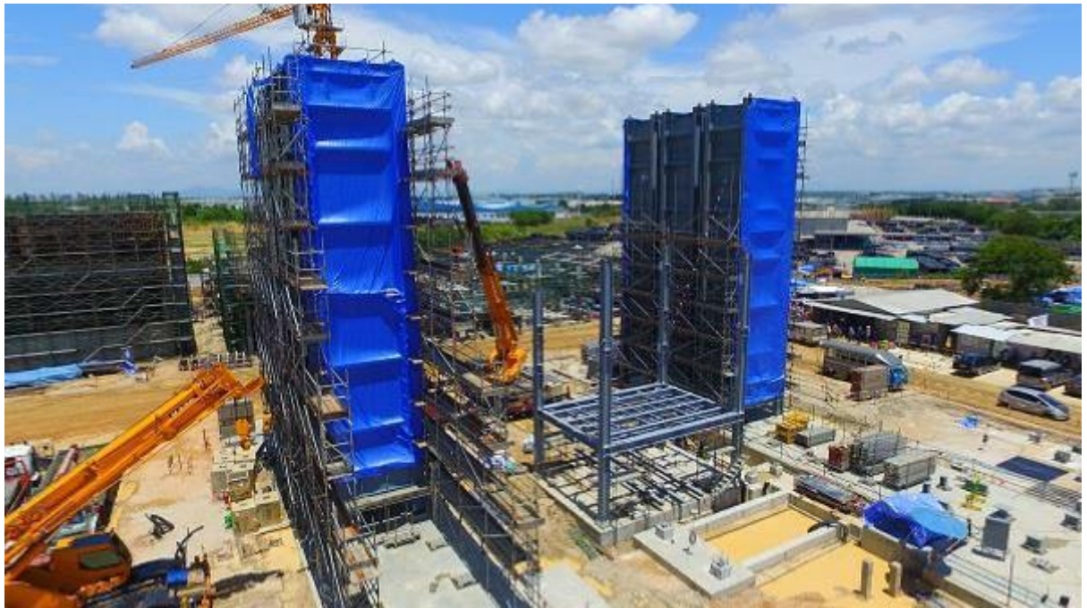
Figure 28 HRSGs installation (Project A monthly reports)
