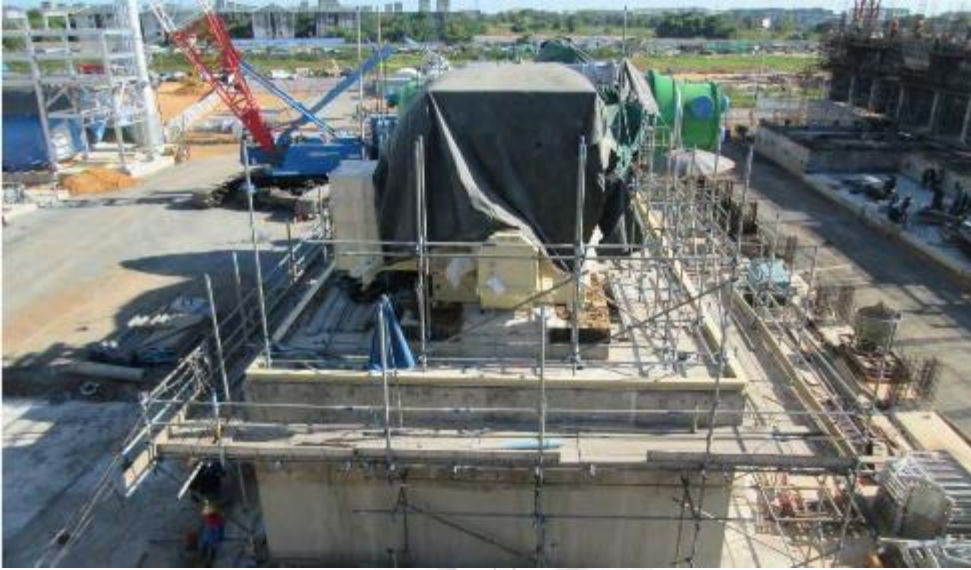
Figure 30 Steam turbine installation (Project C monthly reports)
