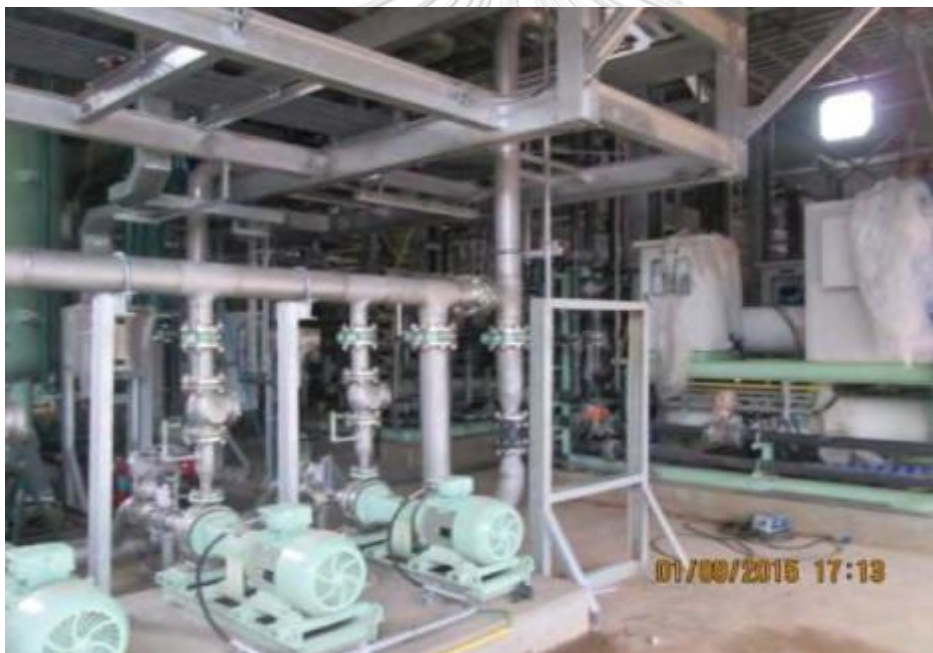
Figure 38 Demineralized water system installation (Project C monthly reports)
