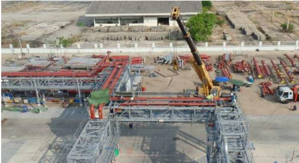
Figure 39 Piping system installation (Project B monthly reports)
