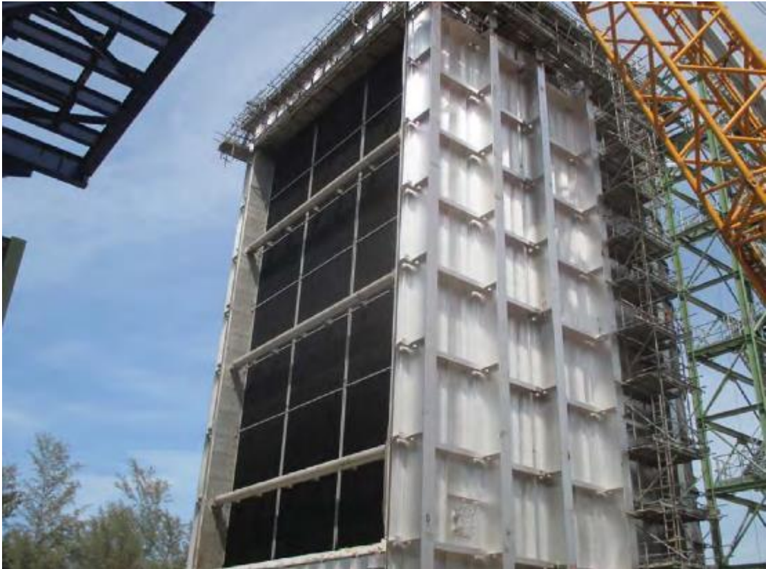
Figure 29 HRSGs installation (Project D monthly reports)
