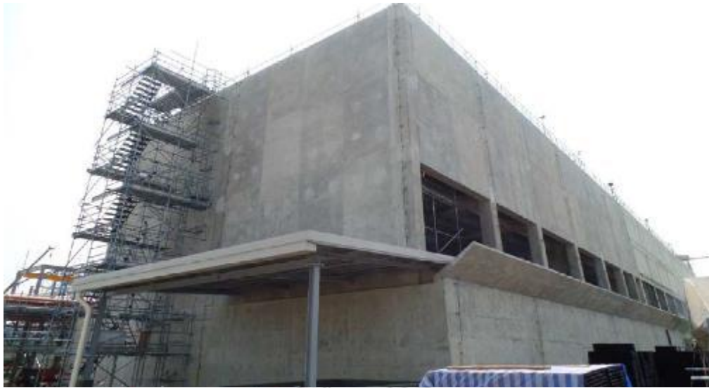
Figure 33 Cooling tower installation (Project B monthly reports)
