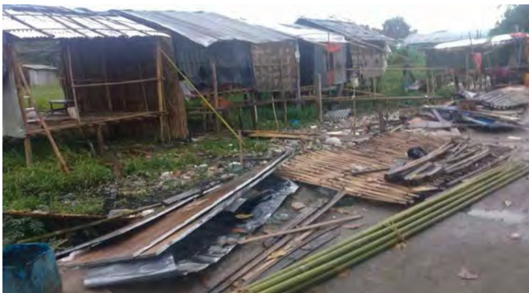
Photo 4. Informal settlement on government land
