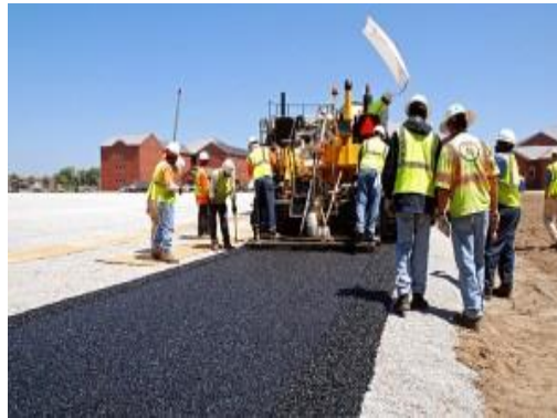
Figure 2.16 Hot mix asphalt construction [35].
