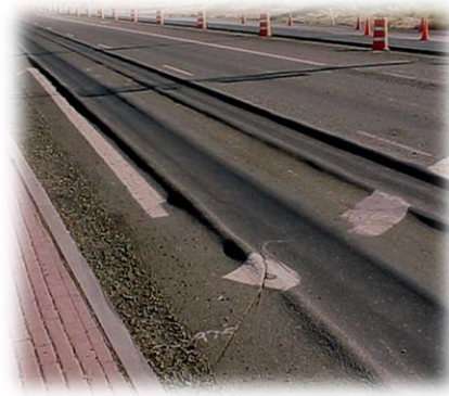
Figure 2.12 Rutting deformation [31].
