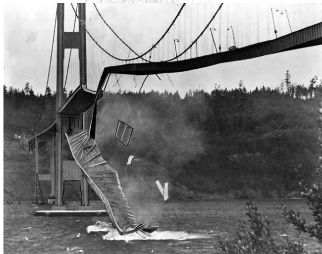
Figure 1. The collapse of Tacoma Narrow Bridge.
