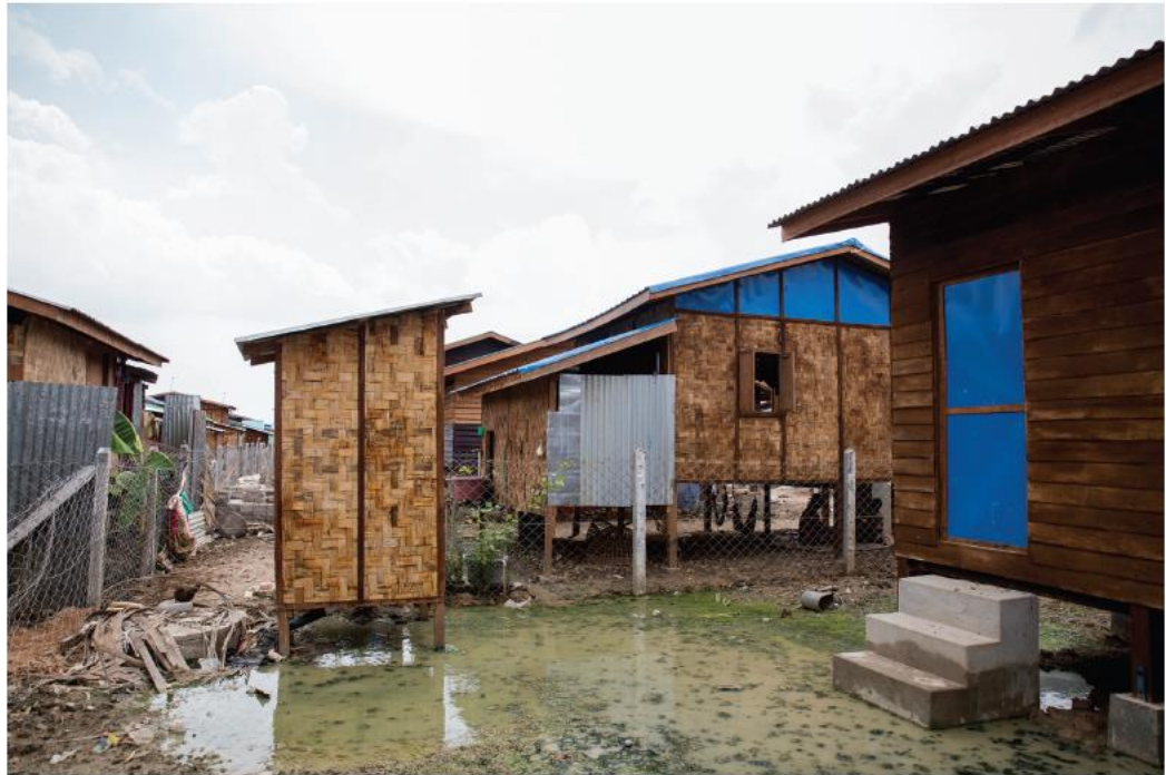
Figure 5 The flooding in the resettlement site of the Phase 1 of Thilawa SEZ Source: EarthRights International. (2014). Analysis of EIA for Phase I of Thilawa SEZ.
