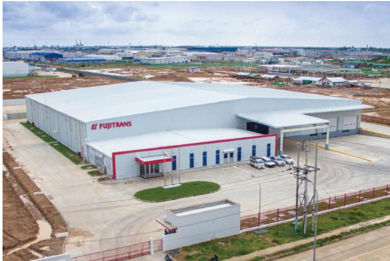
Figure 2 A Warehouse in Thilawa SEZ
