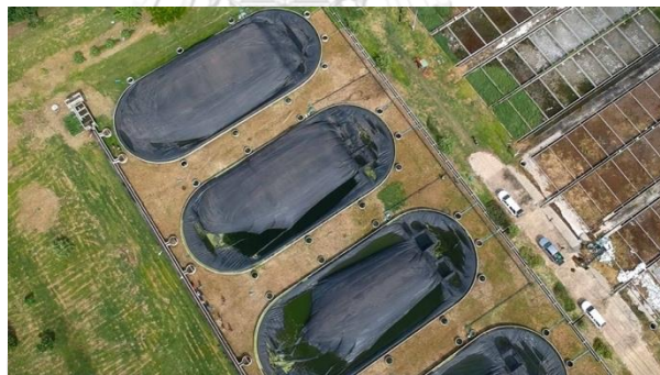
Figure 11: Betagro efficient waste management is carried out through the biogas system.
