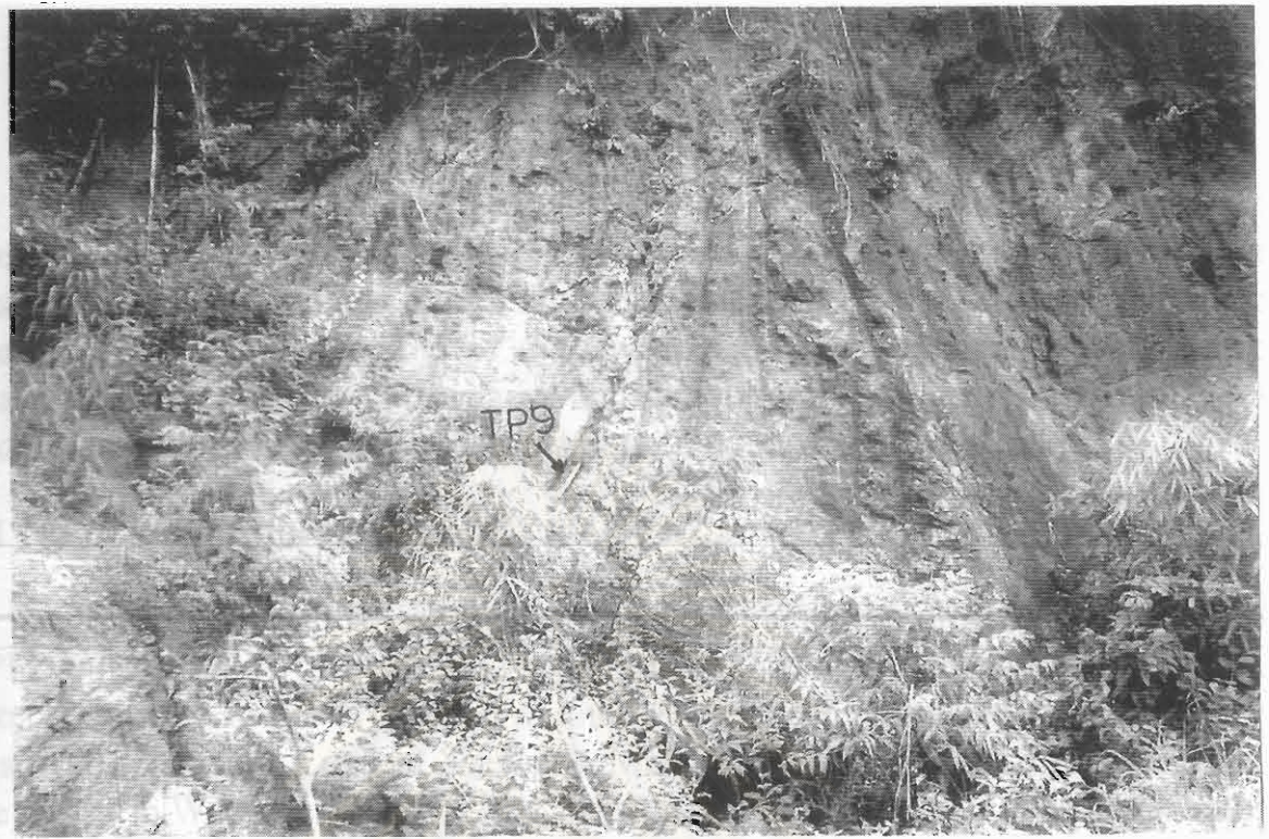
Figure 4.55 Road-cut exposure of weathered yellowish brown to brown, thinly bedded siltstone interbedded with sandstone. Sample no. TP9 was collected from the fault gouge.
