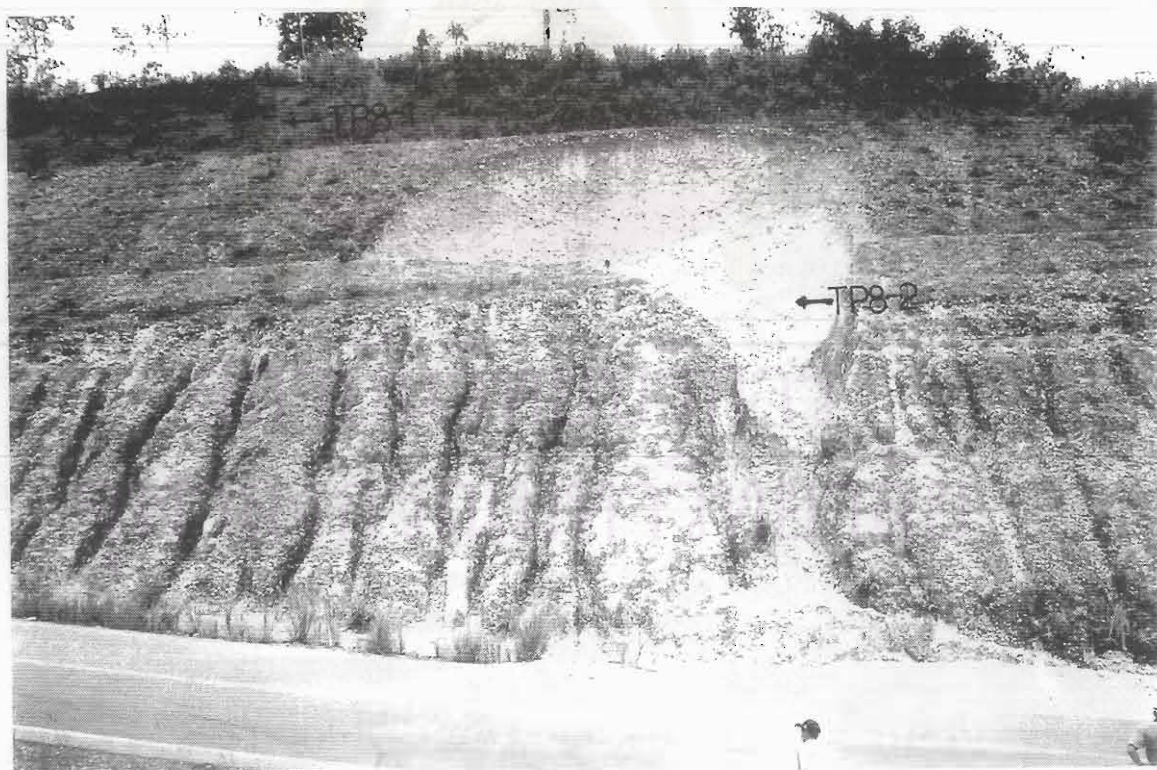
Figure 4.54 Road-cut exposure of gravel beds immediately at the Song Ka Lia River. Samples TP8-1 and TP8-2 were collected from the river gravel bed.
