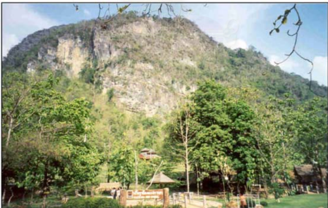
Figure 4.15 Fault scarp observed at eastern side of limestone mountain, indicating youthfulness of the fault in area D.
