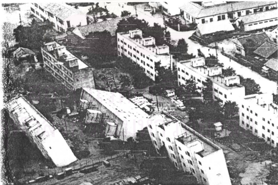
Fig. 2.26. Tilting of apartment buildings, Niigata (1964)
