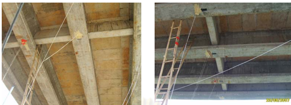
Figure 4.5 Pictures of strain gauges installation
