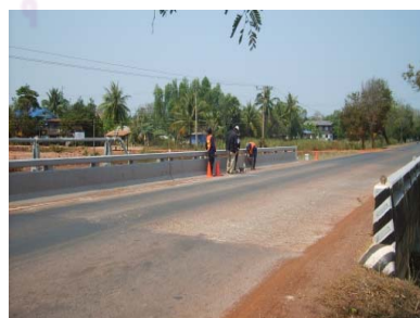
CB6 : Bridge picture, solid parapet type
