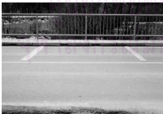
(a) Tape switches axle detector
