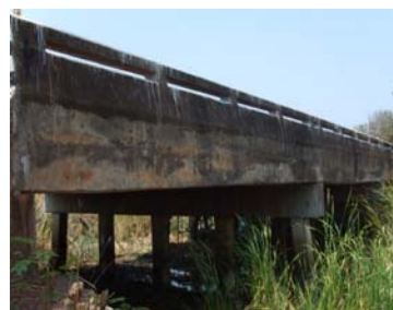
CB6 : Bridge picture, solid parapet type
