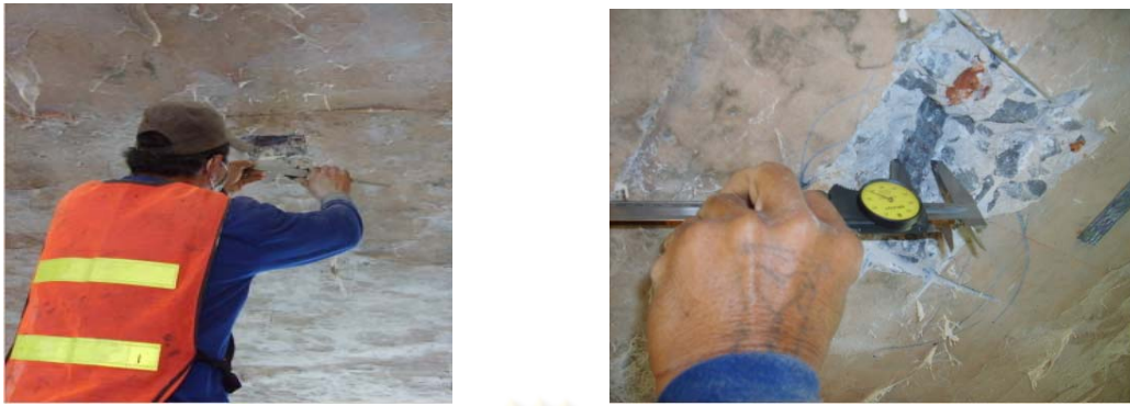
Figure 6.5 Measured the rebar diameter
