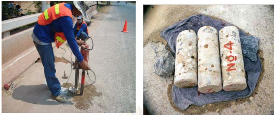
d) Concrete coring
