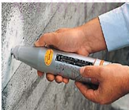
a) Rebound hammer test
