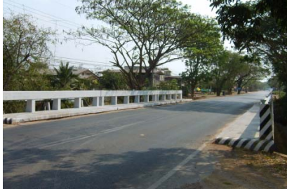
Slab bridges railing barrier type, CB7
