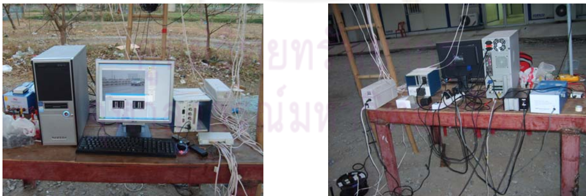
Figure 4.9 Pictures after installation of device completed
