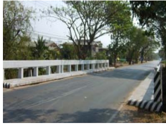
CB7: Bridge picture, railing parapet type
