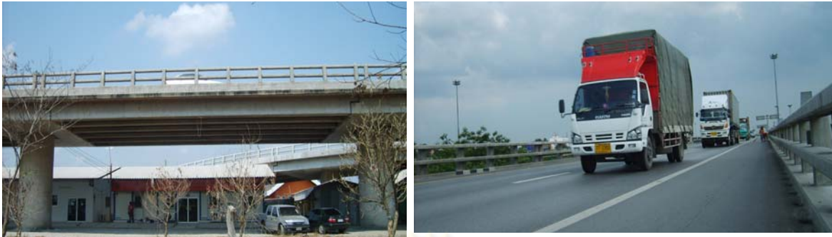
Figure 4.3 Pictures of tested bridge
