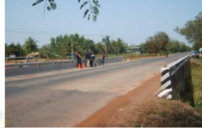
Slab bridges solid barrier type, CB6
