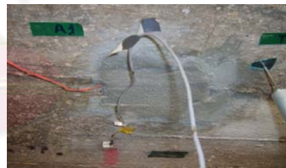
Steel strain gauges embed on bottom of slab, CB6
