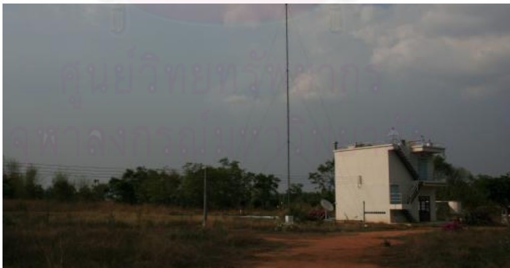
Figure 3.1 The impactors and the meteorological instruments are installed on the roof of the Observatory.
