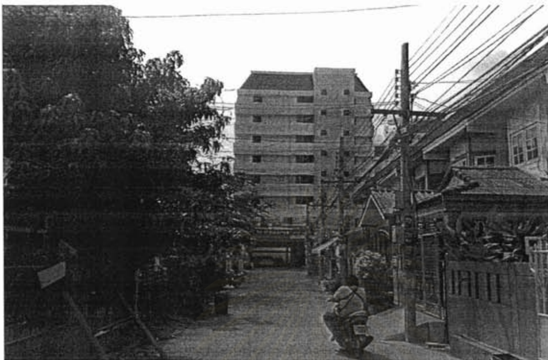
Picture 15 Central Apartment Building
