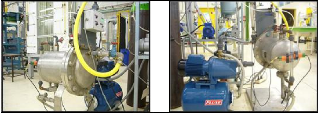
Figure III-12. Photos of the pressurized water system
