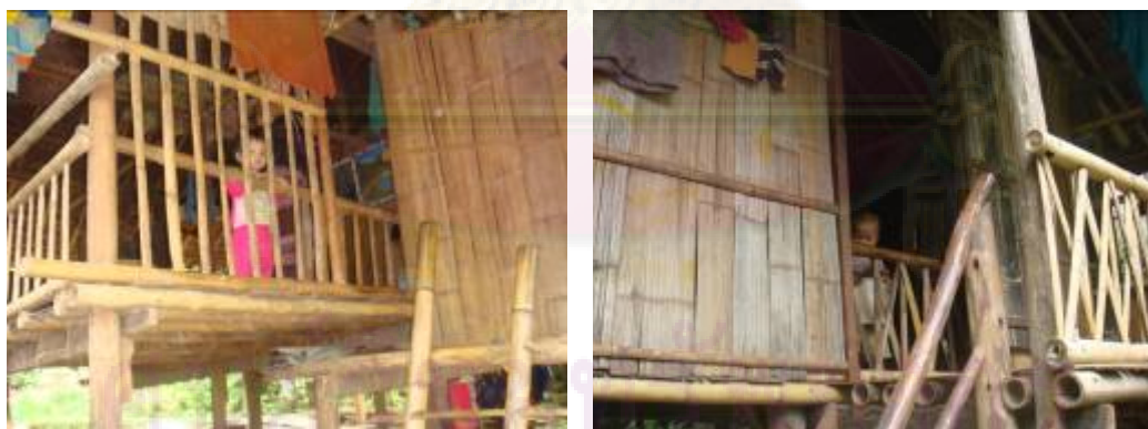
Photo: 15&16 Houses with blocked bamboo bars
