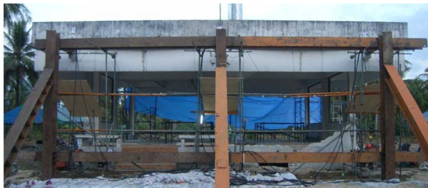
Figure 5-5. Overview of test setup in field load test (front view).
