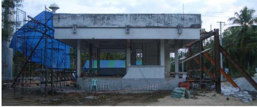
Figure 5-6. Overview of test setup in field load test (side view).
