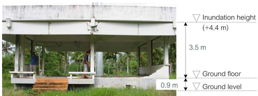
Figure 5-1. Photograph of case study building (front view)
