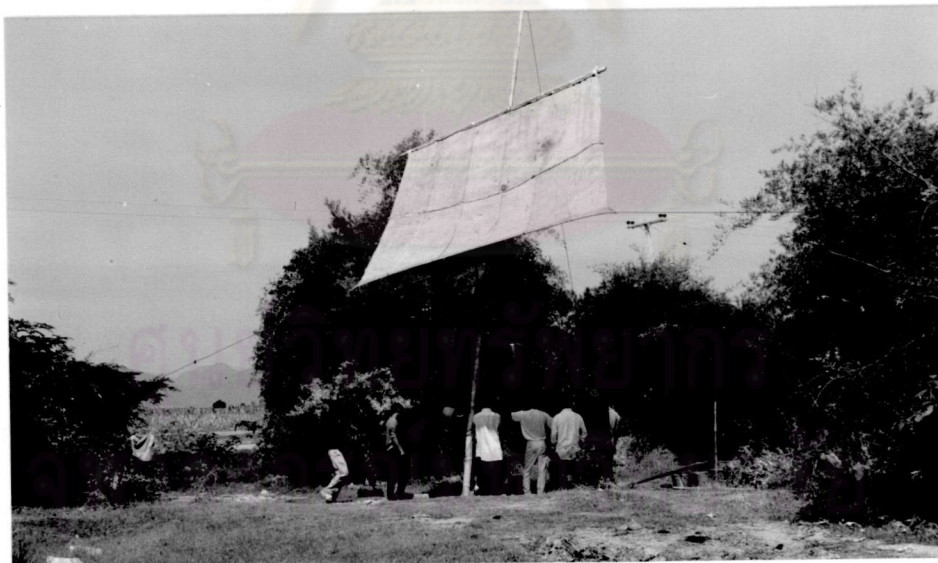
Figure 2.6 Banka drilling is applied to collect samples in the middle part of the area.
