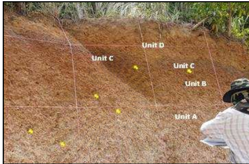
Figure 4.6 Fault (pointed by yellow arrows) with the orientation of N12^{\circ}W72^{\circ}E extending from the bed rock Unit A and ending at the laterite Unit C at the station 54-57 m of the exposure no.1.
