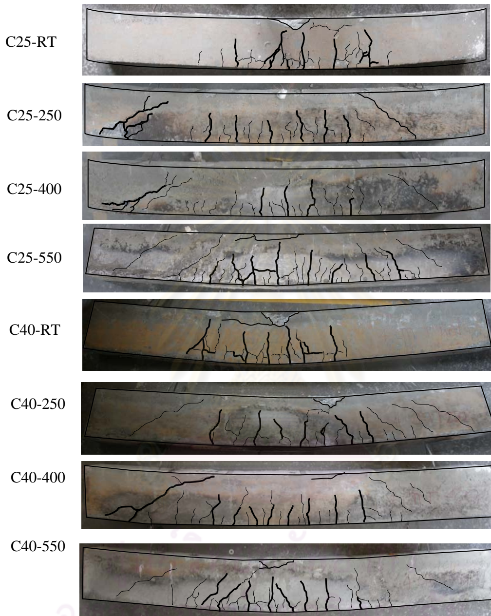
Figure 4.8 Crack patterns of the beam specimens
