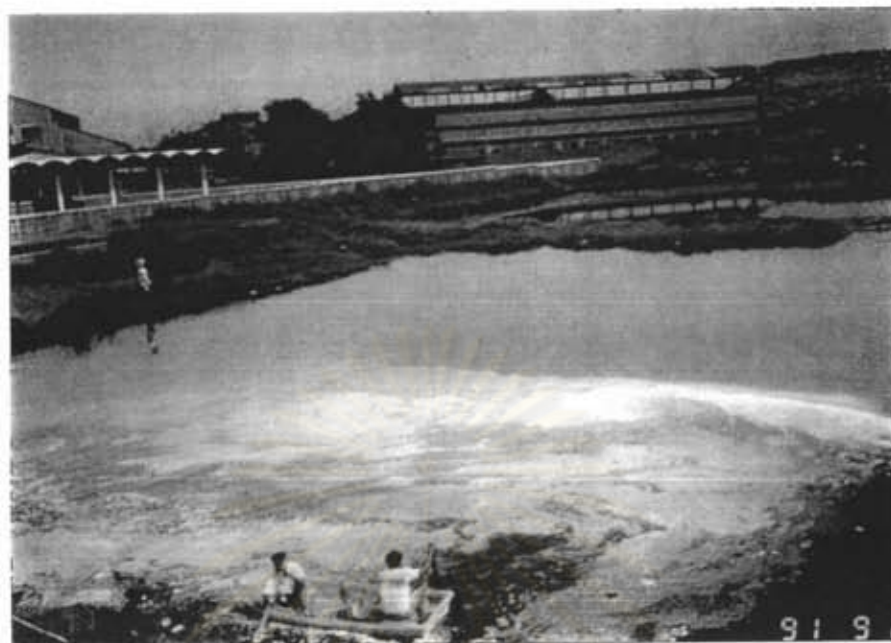
Fig. 3-1 Leachate storage pool at the On-nuch disposal site.
