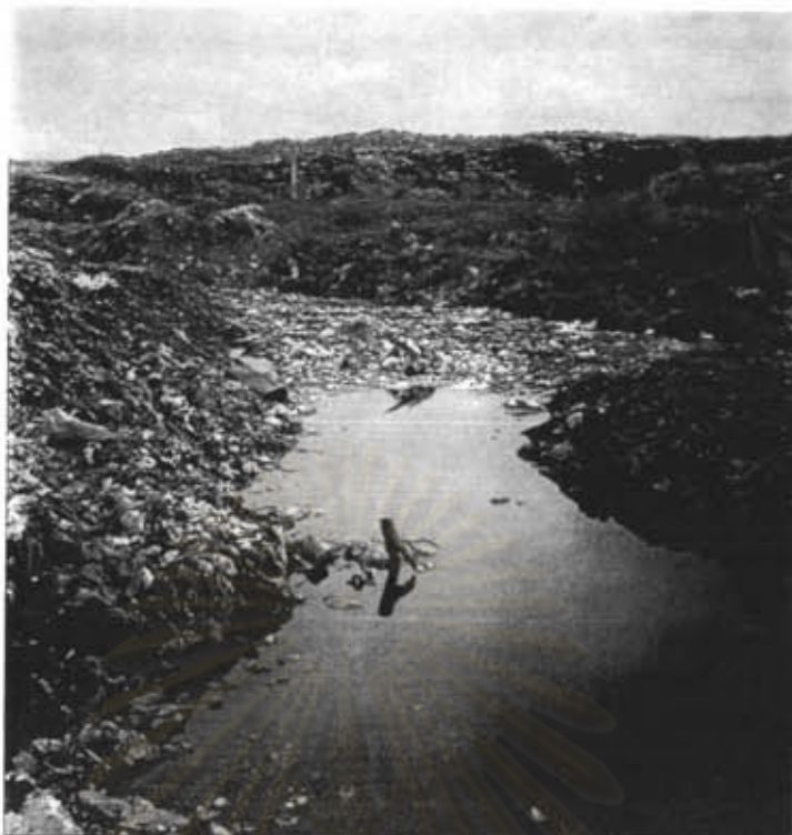
Fig. 3-6 Leachate storage pool at the Nong Kham disposal site.
