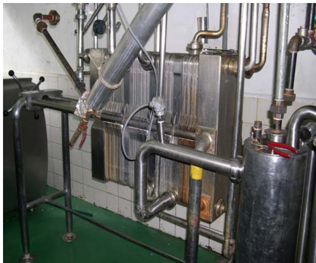
Figure 4.4 Heat exchanger used in pasteurization process
