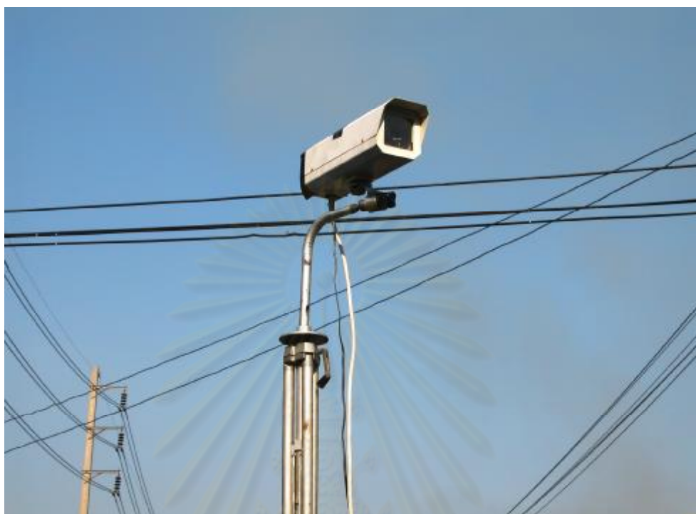
Figure 3.18 Video Camera recorder to record traffic density in the roadside areas.
