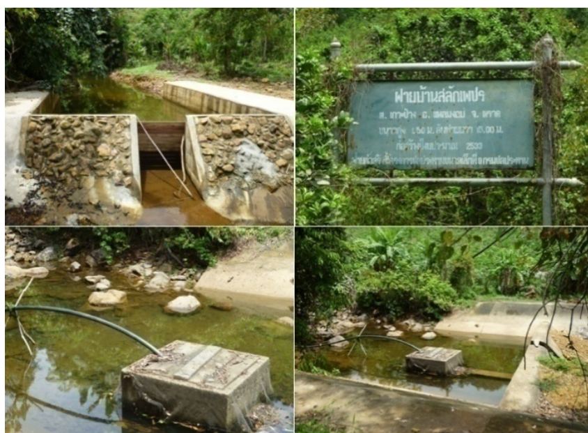
Figure 4.41 The Salak Petch village weir.
